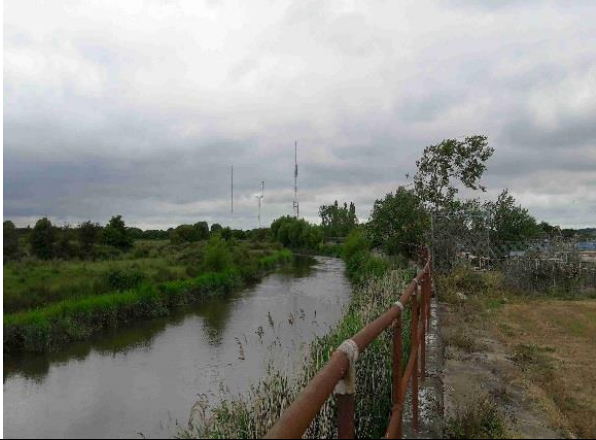
Photo 6: Hard defence on southern boundary of National Grid Energy Transmission Richborough Energy Park (NGR TR3314962077) (June 2017)
