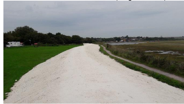
Photo 12: Nemo link onshore overground cable construction in Pegwell Country Park now covered with chalk restoration (August 2017)
