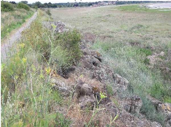
Photo 2: Rock armour sea defence for the historical Cliffsend landfill at Pegwell Country Park (NGR TR3433563145) (June 2017)
