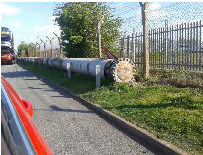
Picture 4 Western end of the pipeline
