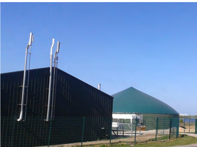
Picture 25 Anaerobic Digester facility within Richborough Energy Park
