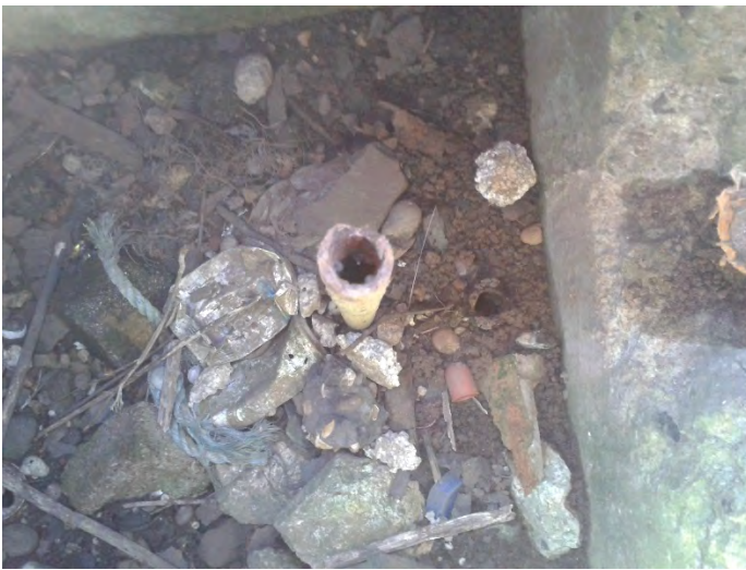
Picture 22 Borehole installation observed on the hoverport tarmac
