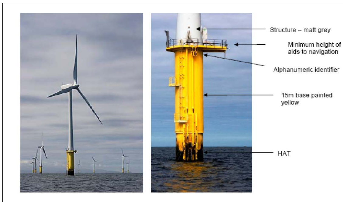
Figure 4: Example of marking a turbine structure 1
