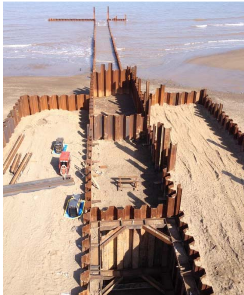
Figure 1.10: Example of an intertidal cofferdam installed using sheet piles.
