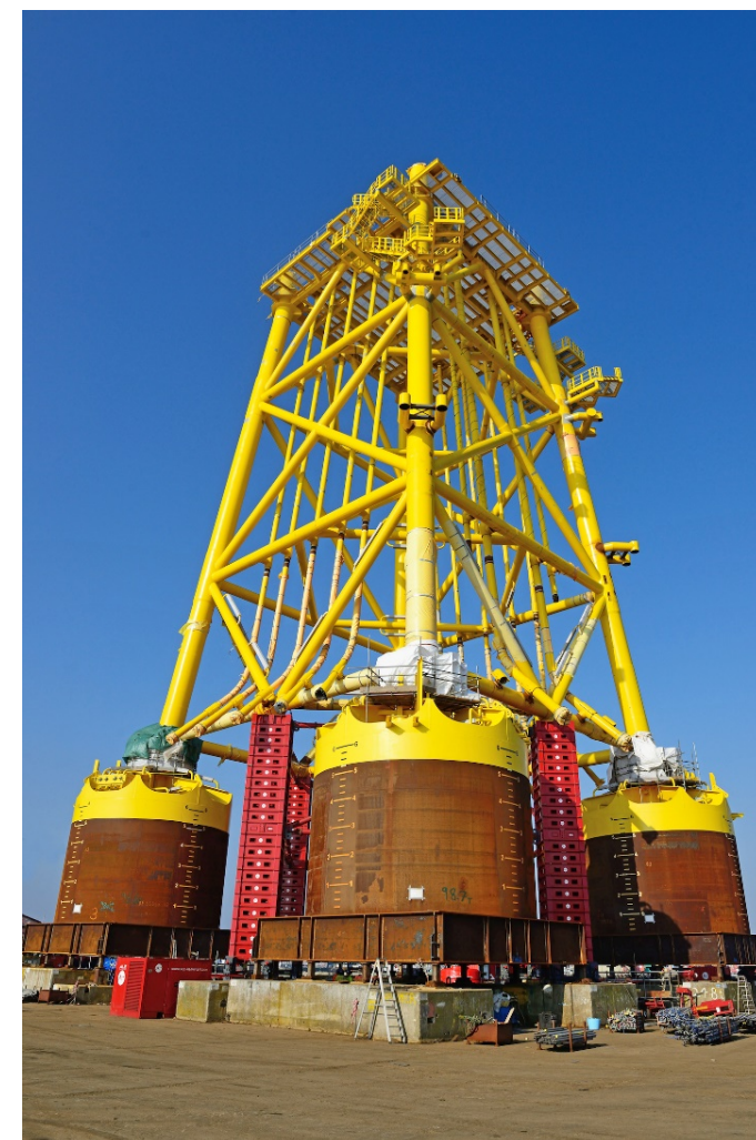
Figure 1.9 Jacket structure with suction caissons
