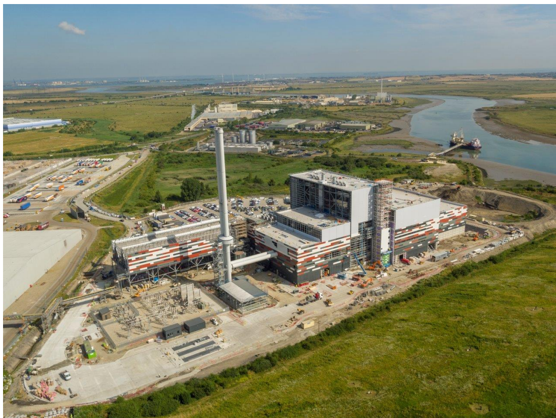
Figure 6.1 – K3 construction progress at July 2019.
