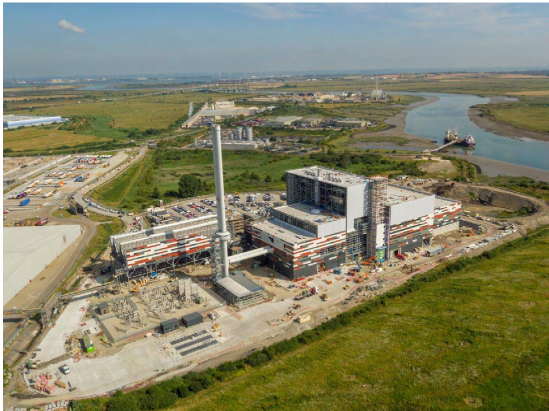
Figure 6.1 – K3 construction progress at July 2019.
