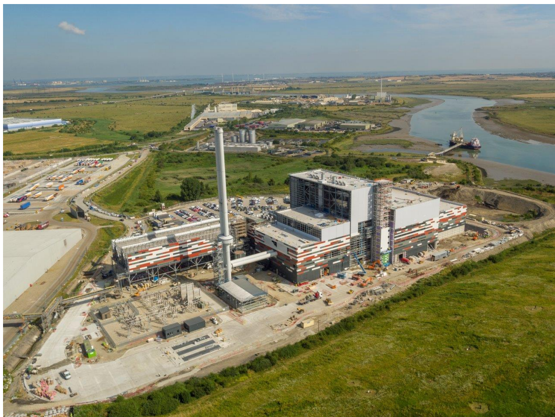
Figure 6.1 – K3 construction progress at July 2019.
