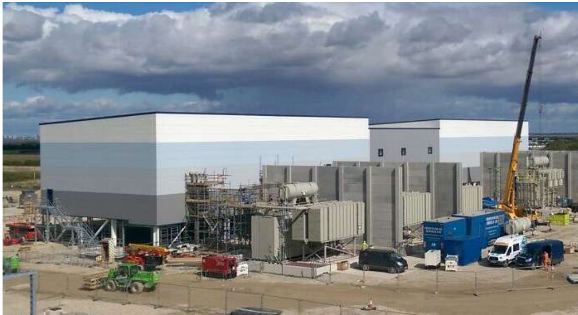
Figure 4.2: Hornsea Project One Onshore Substation during construction
