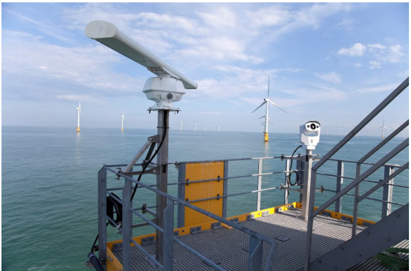
Figure 23. TADS Camera-radar unit installed in Thanet.
