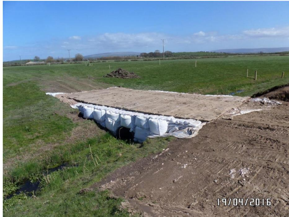
Figure 3.28: A sample flume installation.
