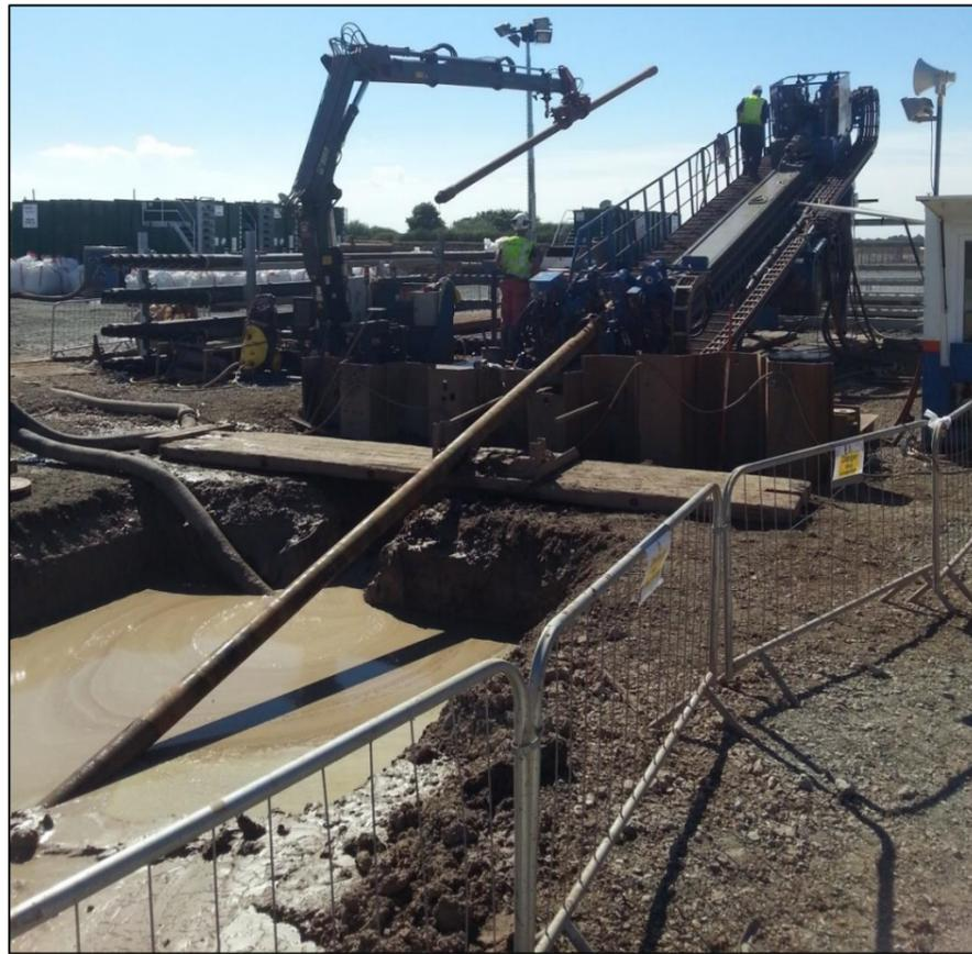
Figure 3.23: HDD rig carrying out landfall works at the Westermost Rough offshore wind farm.
