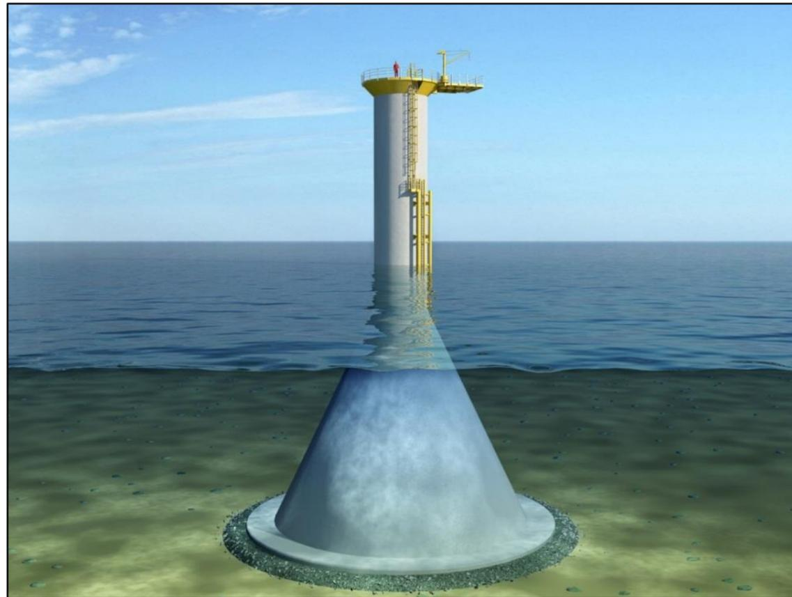
Figure 3.13: A gravity base foundation.
