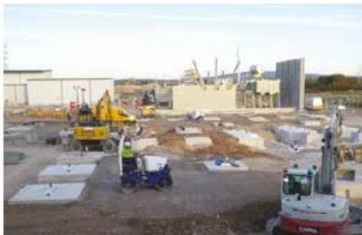
Construction of the substation at Walney Extension Offshore Wind Farm.
