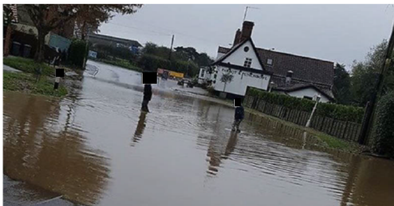
Repeated flooding, due to blocked underground seepage by a housing development in the valley, cut the village of Aldringham in half — this image was taken in 2019; drainage was eventually installed in 2020.
