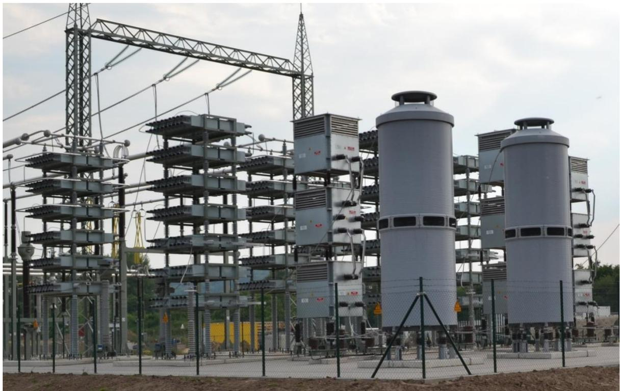
**Figure 1 Capacitor banks split into two to reduce height**
