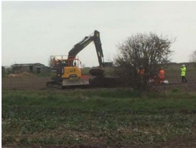
Excavator by stables.
