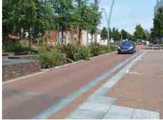
Figure 9.9 Bioretention system, inner ring road around Ashford town centre (courtesy Kent County Council)
