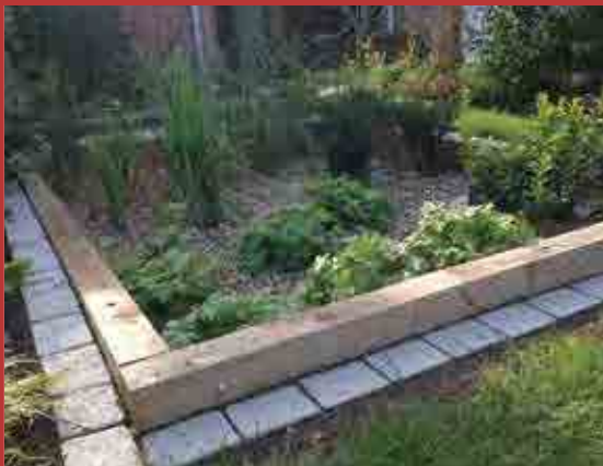
Figure 34.9 A completed rain garden (courtesy Illman Young)
