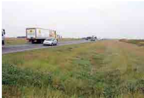
Figure 9.5 Swale and wetland system, A16, Lincolnshire (courtesy EPG Limited)
