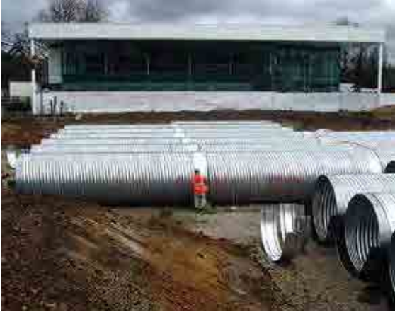
Figure 21.12 Typical corrugated steel tank under construction (courtesy Tubosider UK Limited)
