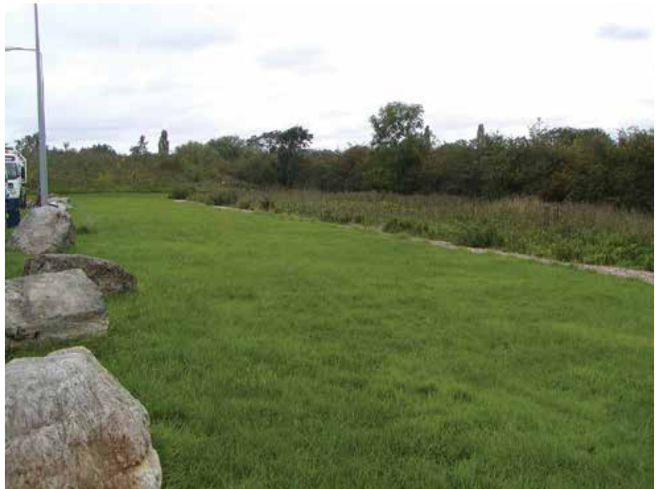
Figure 15.1 Filter strip at motorway services draining to filter drain, Hopwood (courtesy Illman Young)
