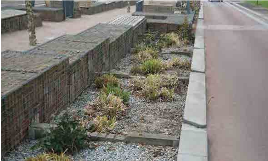
Figure 10.13 Rain garden with weirs to control flows on sloping site in Ashford, Kent (courtesy EPG Limited)
