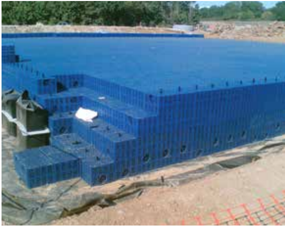
Figure 21.2 Structural frame being constructed (courtesy EPG Limited)
