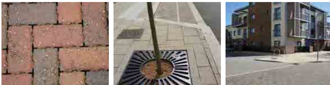
Figure 10.2 Pervious surfaces (courtesy Interpave)
