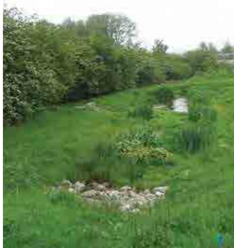
Figure 23.11 Balancing pond with marginal wetland treatment zone, Hopwood Park motorway services, M42, Worcestershire
