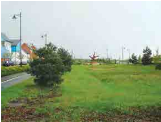
Figure 13.6 Large infiltration basins, Ipswich (courtesy Graham Fairhurst)
