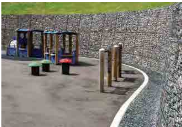
Figure 16.3 Filter drain with exceedance event managed within play area, Exwick, Devon (courtesy Robert Bray Associates)
