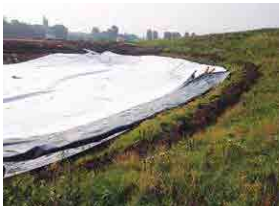
Figure 30.3 Installation of pond liner with protection fleece (courtesy Stormwater Management)
