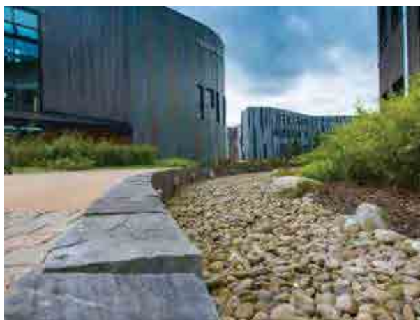
Figure 28.5 Timber sleeper edging with gaps, University of York (courtesy Arup/Giles Rocholl Photography)
