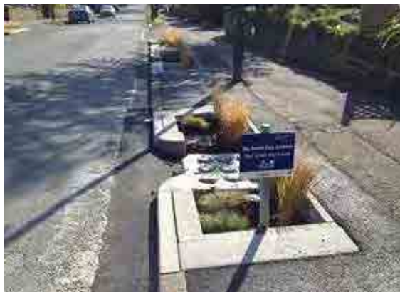
Figure 5.5 Rain garden, Ribblesdale Road, Nottingham (courtesy Environment Agency)
