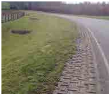
Figure 8.8a Check dams in a swale, Oxfordshire (courtesy EPG Limited)
