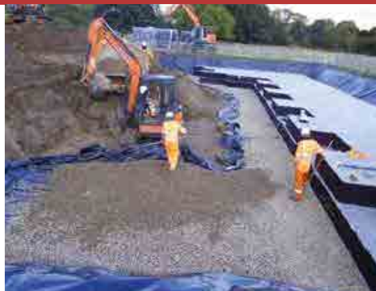
Figure 35.2 Dulwich Park geocellular storage tank during construction (courtesy Project Team)
