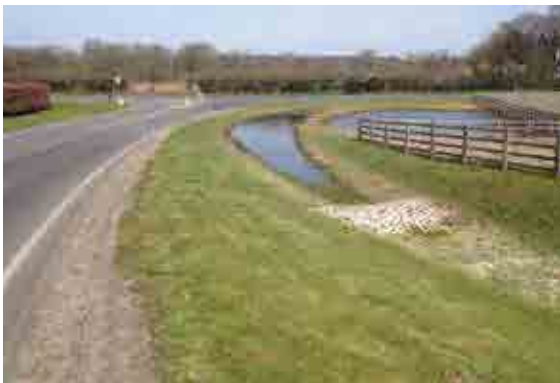
Figure 9.4 Swale on a steeply sloping road, Oxfordshire (courtesy EPG Limited)
