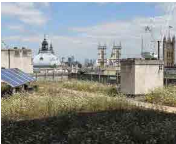
Green roof (courtesy Green Roof Consultancy)
