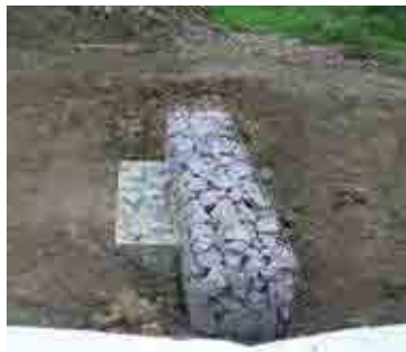
Figure 8.8b Check dam in a swale during construction, Lincoln (courtesy Lincolnshire County Council)
