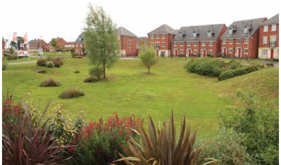
Figure 22.1 Detention basin with landscape design providing attractive amenity space, Hamilton, Leicester
