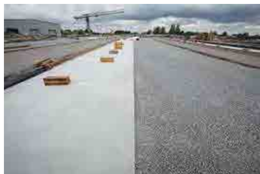
Figure 30.1 Construction of a drainage layer (courtesy EPG Limited)
