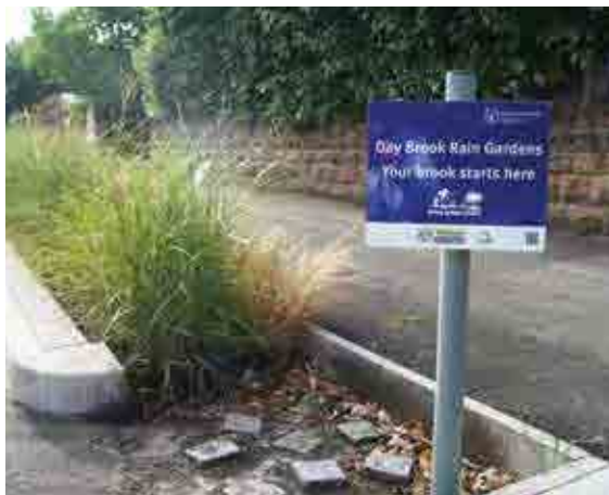
Figure 18.11 Example of a bioretention system with a simple sediment forebay, Nottingham (courtesy Environment Agency)
