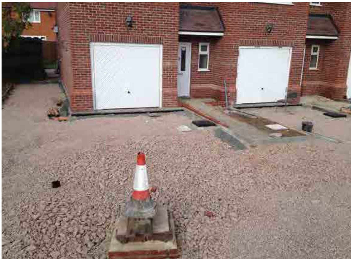
Figure 31.3 Concrete block permeable paving being constructed at the end of the project (courtesy EPG Limited)
