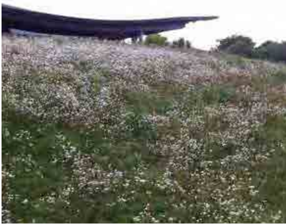
Figure 12.2 The Savill Garden extensive green roof
