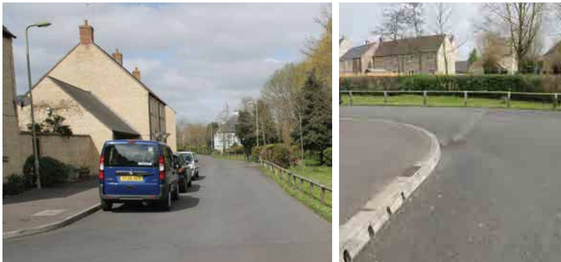
Figure 9.16 Kerb drains and channel connected to swale (courtesy EPG Limited)
