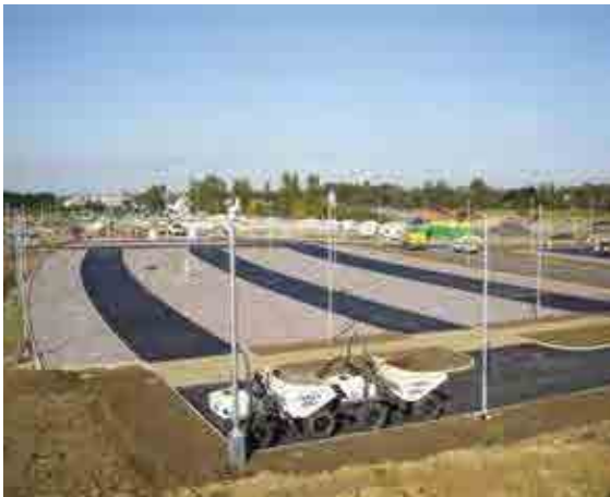
Figure 20.1 Park and ride scheme on the outskirts of Cambridge using concrete block permeable paving (courtesy EPG Limited)
