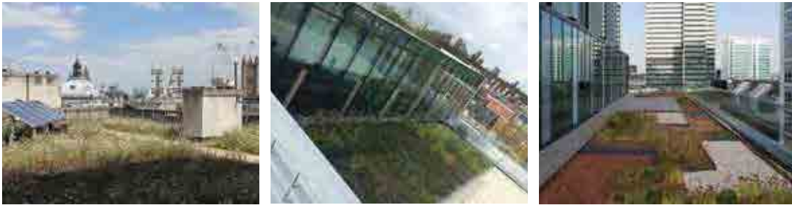
Figure 10.8 Green roofs (courtesy Sky Garden, Arup)
