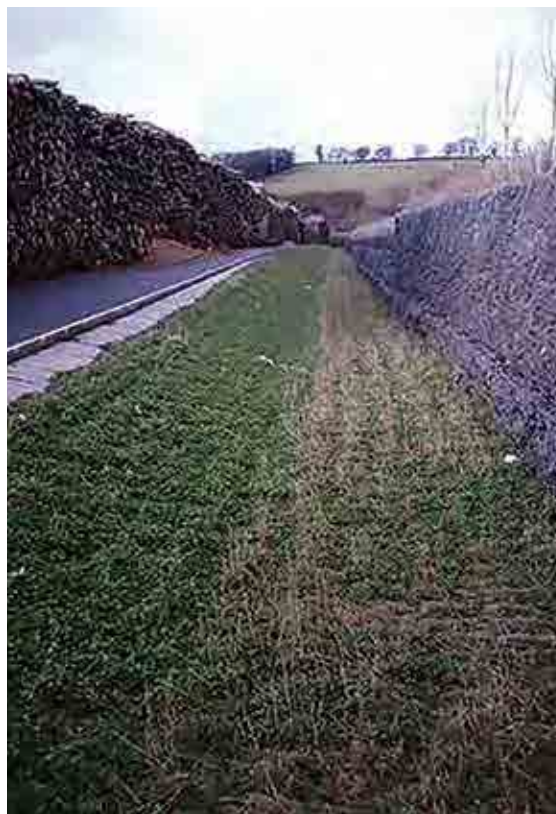
Figure 17.6 Swale with vertical side (courtesy EPG Limited)
