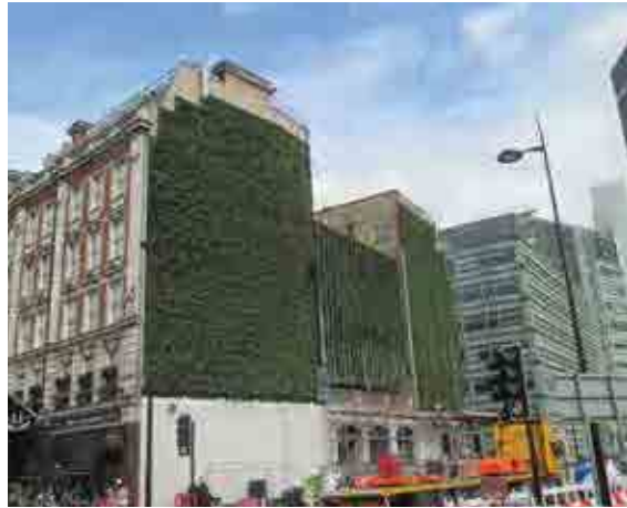
Green wall (courtesy Green Roof Consultancy)
