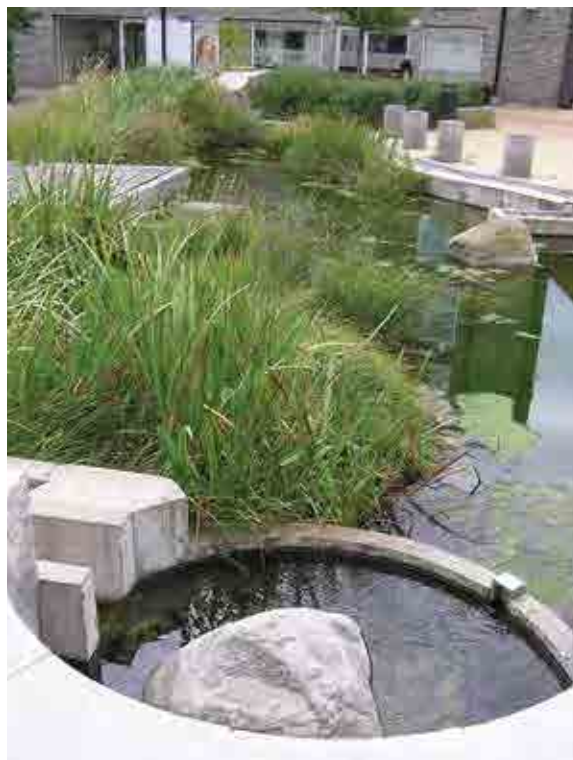
Figure 23.7 Pond with baffles and islands, Augustenborg, Sweden
