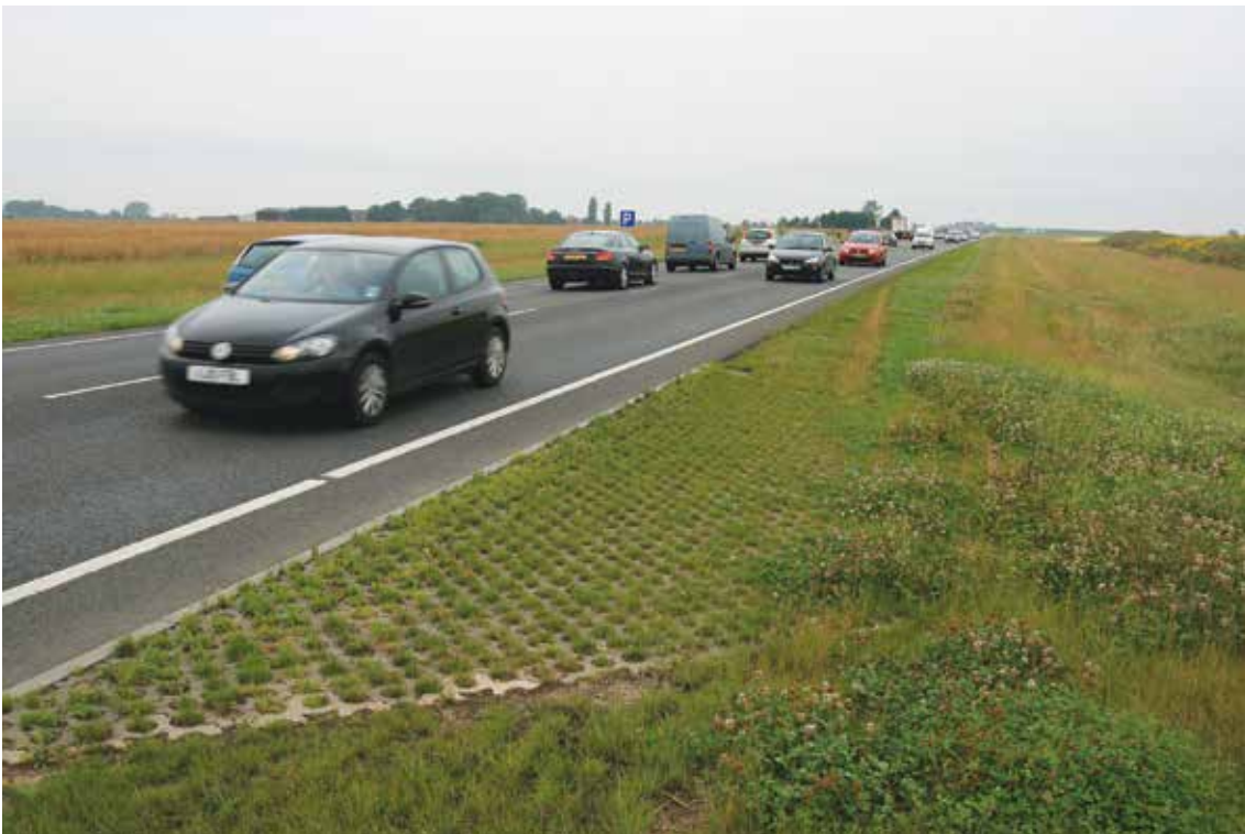
Figure 9.3 Swale and wetland systems with reinforced grass used in less trafficked areas such as laybys and field access points, A16, Lincolnshire (courtesy EPG Limited)
