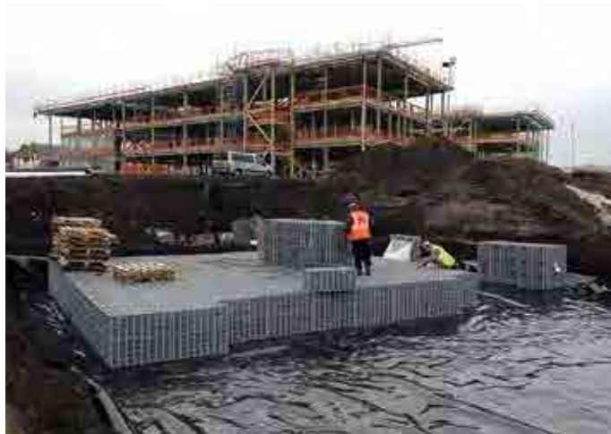
Figure 21.1 Geocellular storage system under construction (courtesy Polypipe Limited)
