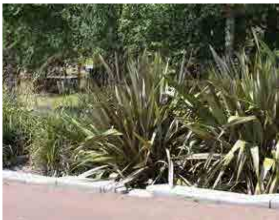
Bioretention system (courtesy Essex County Council)
