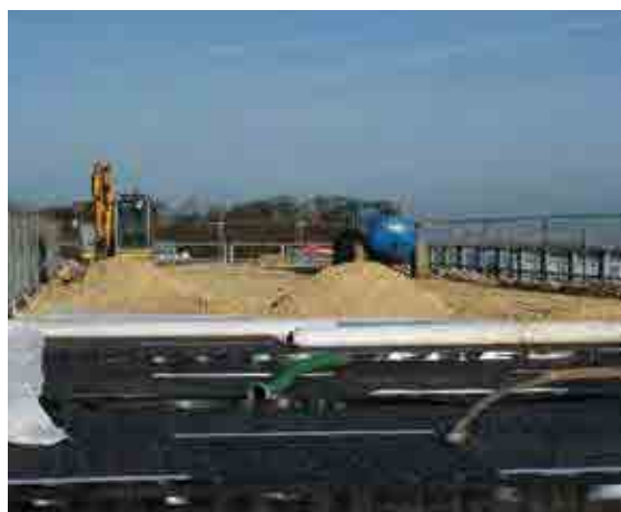
Figure 20.11 Construction of attenuation and irrigation system used below equestrian surfacing (courtesy Andrew Bowen)
