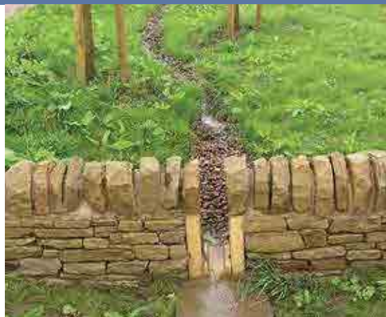
Figure 6.2 Conveyance component (courtesy Sheffield City Council)
