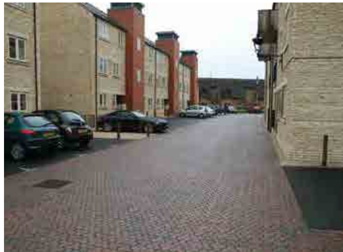
Figure 8.2 Unlined permeable pavement on a contaminated site, Stamford, Lincolnshire (courtesy EPG Limited)
