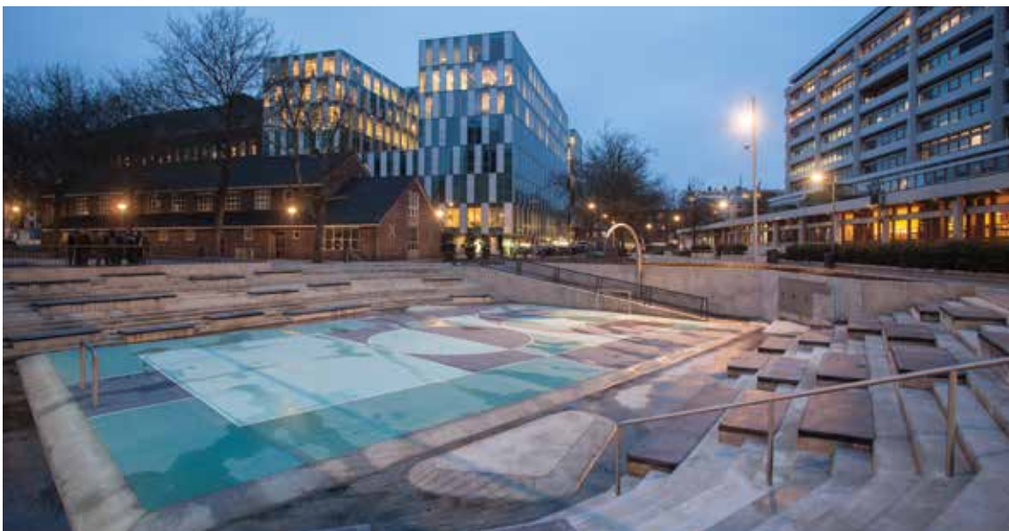
Figure 22.5 Example of urban hard surfaced off-line detention basin with geometric design to enhance amenity use, Rotterdam, the Netherlands (courtesy pallesh+azarfane)
