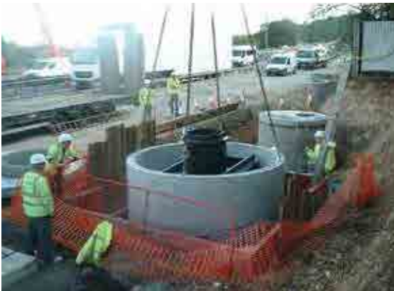
Figure 9.10 Installation of vortex separator, M25 (courtesy Hydro International)
