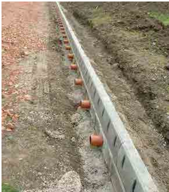
Figure 20.8 Macro pervious pavement under construction in the Midlands – kerb drain collector/pollution trap with connectors before placing diffusers and permeable sub-base to the left (courtesy Phil Tomlinson)
