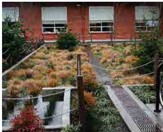
Figure 18.12 Bioretention system inundated during heavy rain, showing submerged forebay (front left), Portland, Oregon (courtesy Environmental Services, City of Portland)
