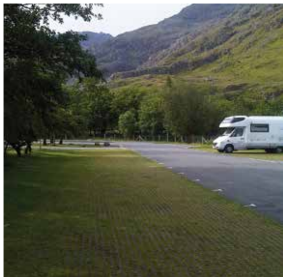
Figure 20.5 Concrete grids in a park and ride overflow car park, Gwynedd (courtesy EPG Limited)
