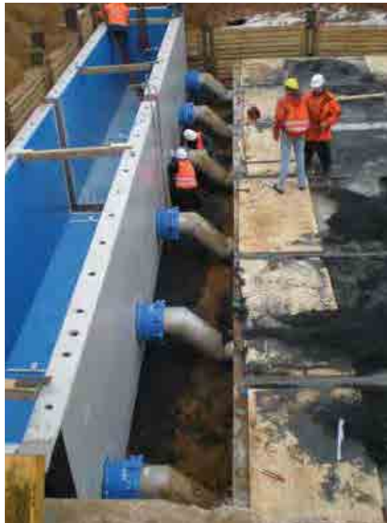
Figure 14.9 Large oil separator under construction (courtesy ACO Limited)
