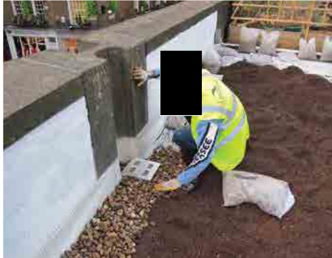
Figure 12.15 Installing a green roof outlet with surface overflow (courtesy Clare Dinham)
