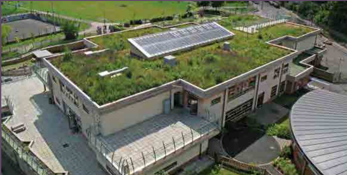
Figure 12.13 Sharrow School green roof (courtesy The Green Roof Centre)
