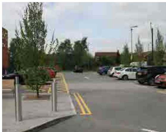
Figure 20.7 Retail development car park with porous concrete, High Wycombe (courtesy EPG Limited)
