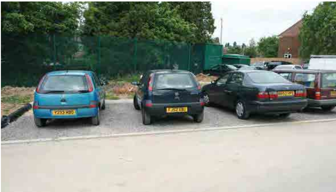
Figure 31.4 Temporary surface over permeable sub-base in parking bays (geotextile and hardcore) (courtesy EPG Limited)
