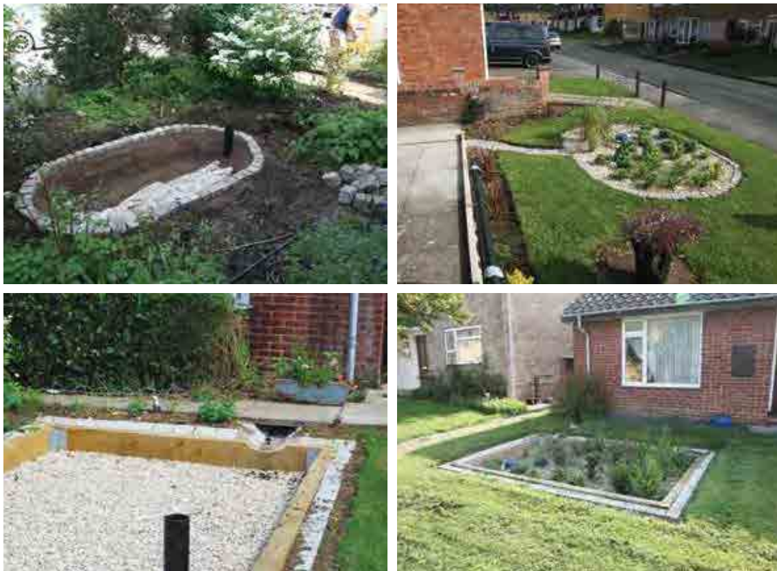
Figure 18.3 Examples of rain gardens under construction and planted, Cheltenham (courtesy EPG Limited and Illman Young)
