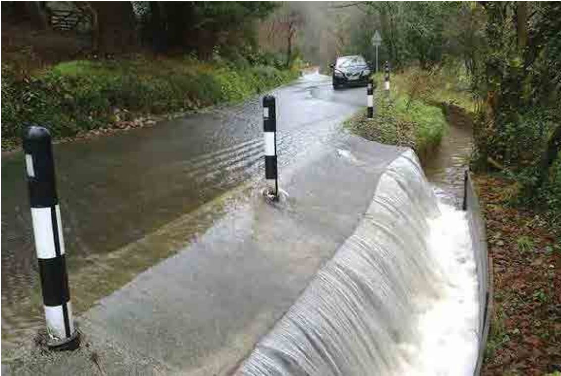
Figure 9.19 Highway acting as a flood pathway in an exceedance event (courtesy Simon Jeffrey)
