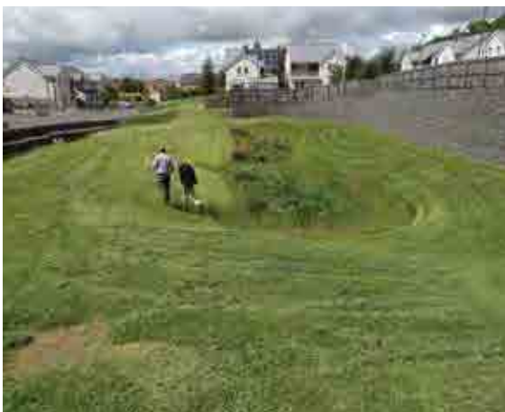
Figure 22.3 Detention basin serving a housing estate, Stirling (courtesy Abertay University)
