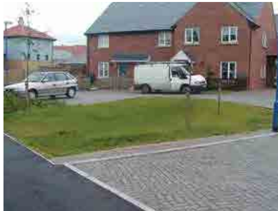
Figure 13.7 Small infiltration basin, Cambourne (courtesy Illman Young)
