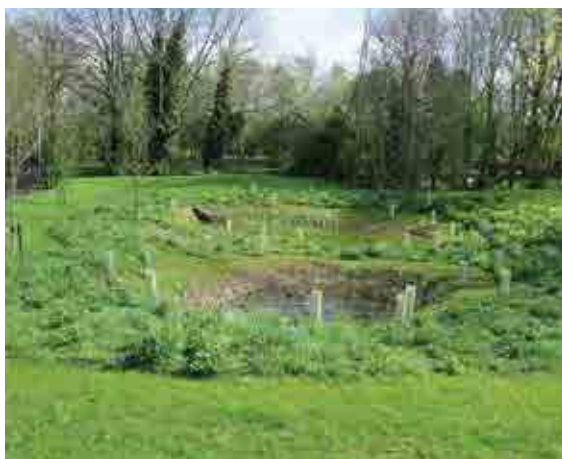
Figure 6.8 Infiltration basin with wildflower turf and grass seeding, Victoria Park Health Centre, Leicester (courtesy DSA Environment and Design)
