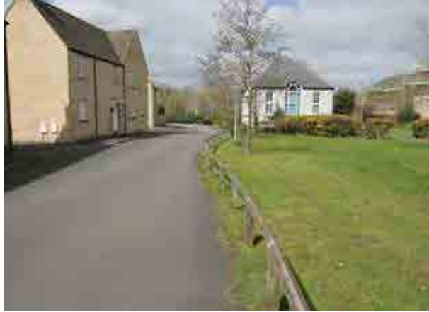
Figure 8.5 Shallow swale on a site with shallow groundwater, Witney, Oxfordshire (courtesy EPG Limited)
