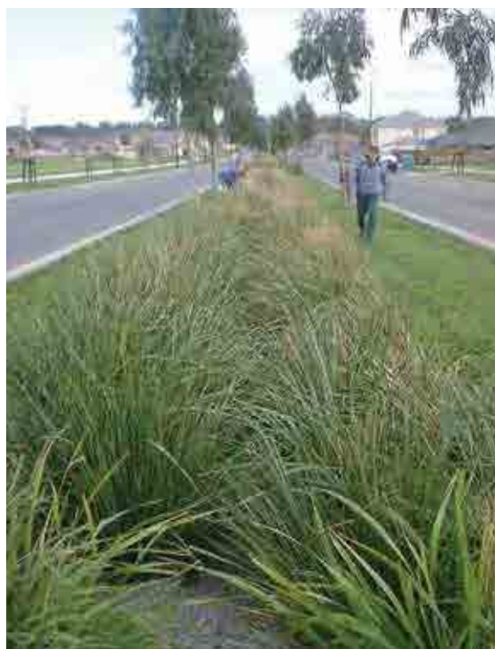
Figure 18.7 Bioretention swale (courtesy Derwent Estuary)
