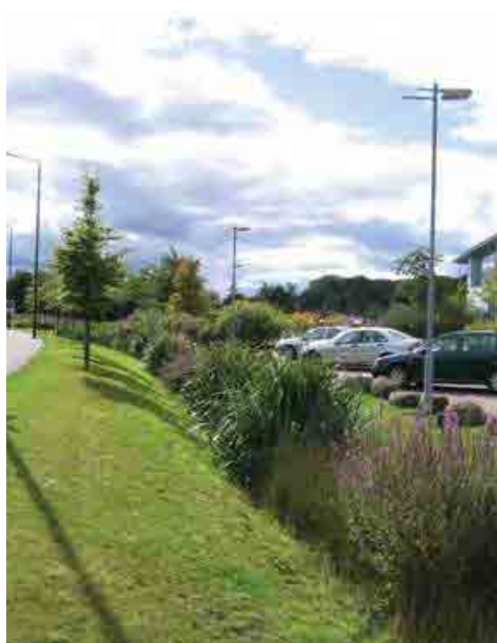
Figure 17.11 Linear wet swale, Junction 4 M8, West Lothian
