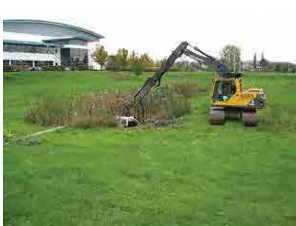
Figure 32.2 De-silting (courtesy Bedford Group of Drainage Boards)
