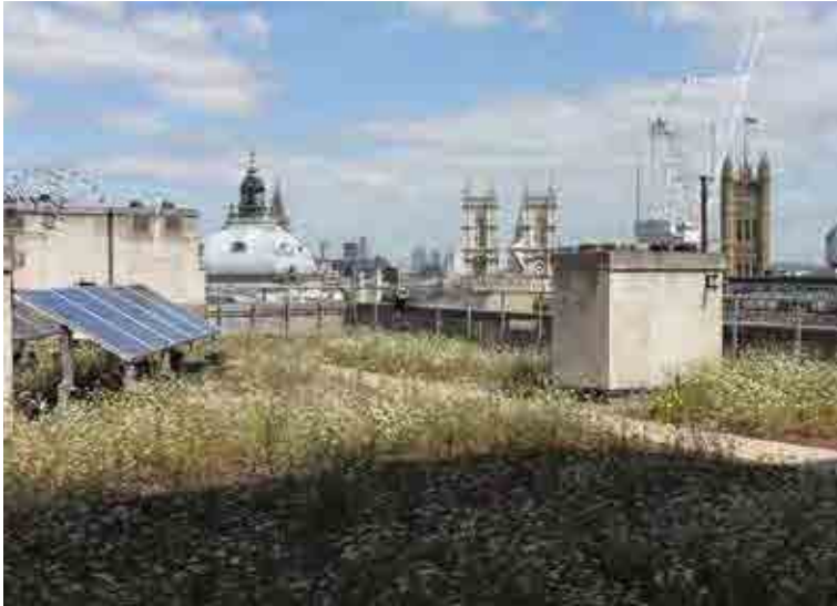
courtesy Green Roof Consultancy
