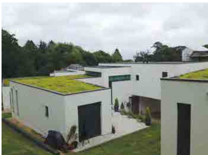
Figure 12.5 Domestic green roofing, Swansea (courtesy Sky Garden)
