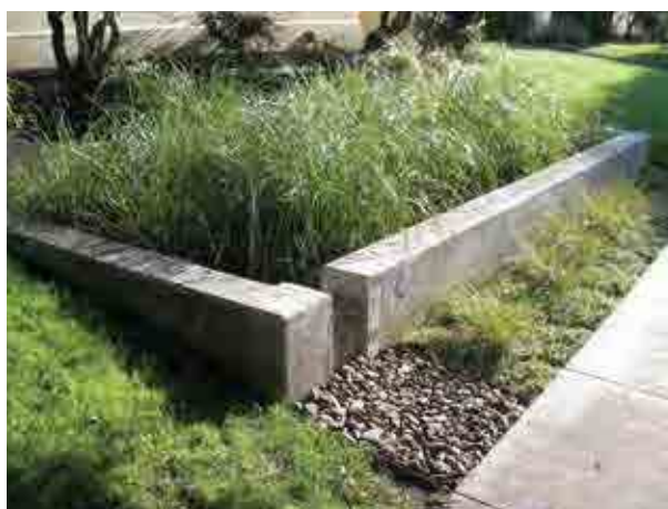
Figure 18.18 Example of a simple rain garden overflow, Portland (courtesy Illman Young)
