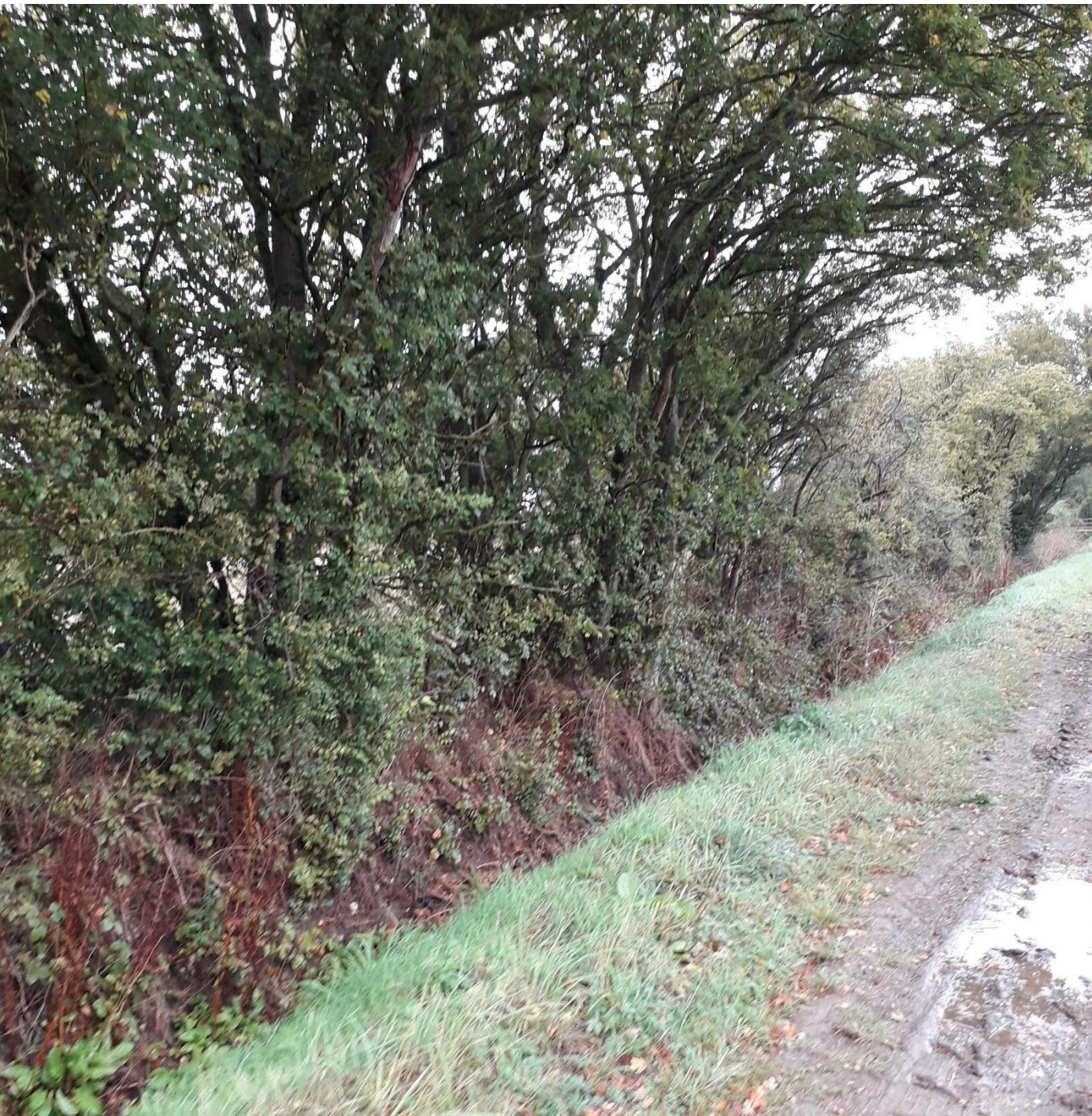
Photo 8 Looking north. Ditch and hedge lining track
