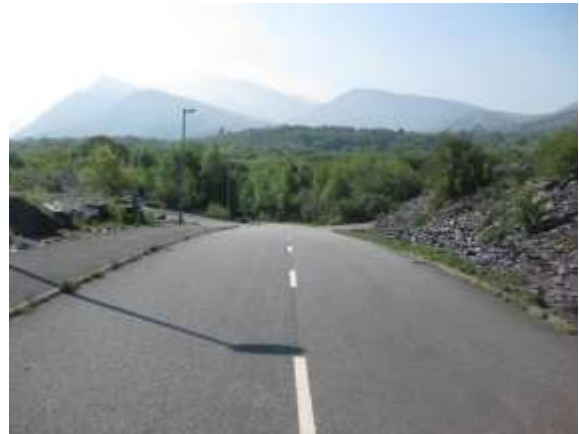
16. View north on to newly constructed highway, with footway to the west and loose material to the east.
