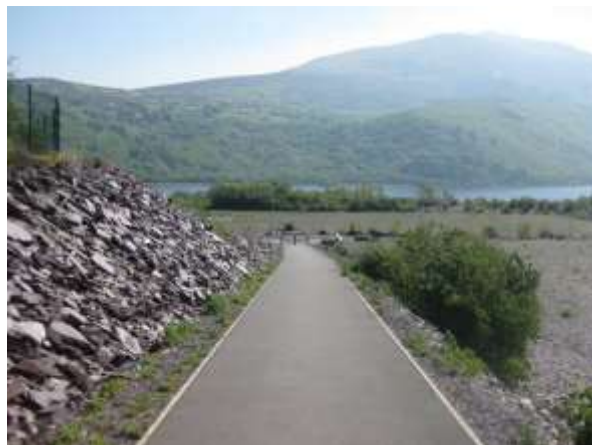
3. View south on to newly constructed footway.
