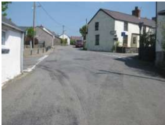
47. Groeslon crossroads looking north features white lining at the junctions but no centre-lines. The highway is closely bound by residential dwellings and is of reasonable condition. There is a paved area to the north west of the junction which is protected by short bollards.
