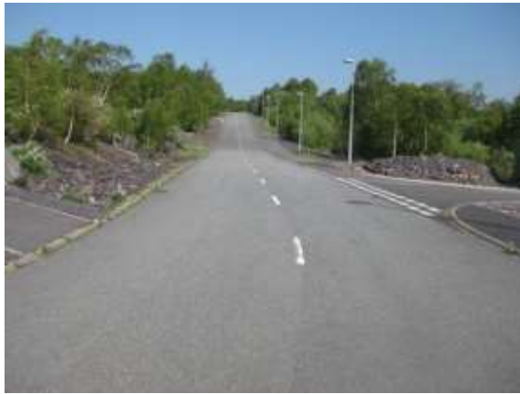
15. View south on to newly constructed highway, with priority junction to the east.
