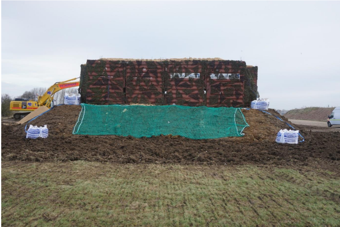
Figure 1: Typical EOD Facility
