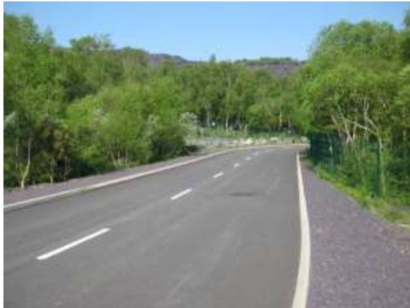
7. View north - Loosely surfaced footway at either side of newly constructed highway.
