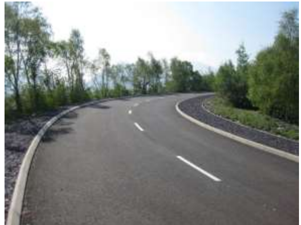
6. View south at newly constructed industrial road - Loosely surfaced footway at either side of newly constructed highway
