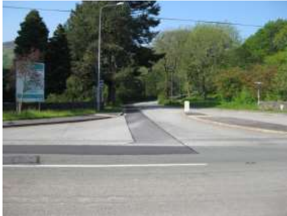
27. View south on to priority junction leading to Glyn Rhonwy. Highway shows signs of resurfacing and is bound by street lighting to the west. Central reservation with traffic island is present.
