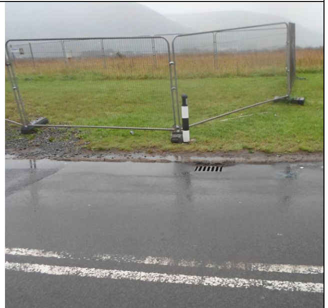
Photograph 4: Onsite road with drains
