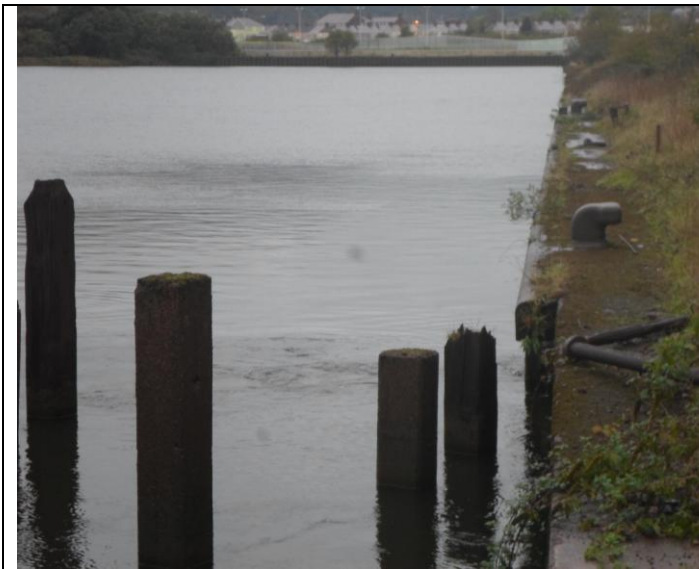
Photograph 5: Discharge point for current cooling towers and boilers to Port Talbot Dock
