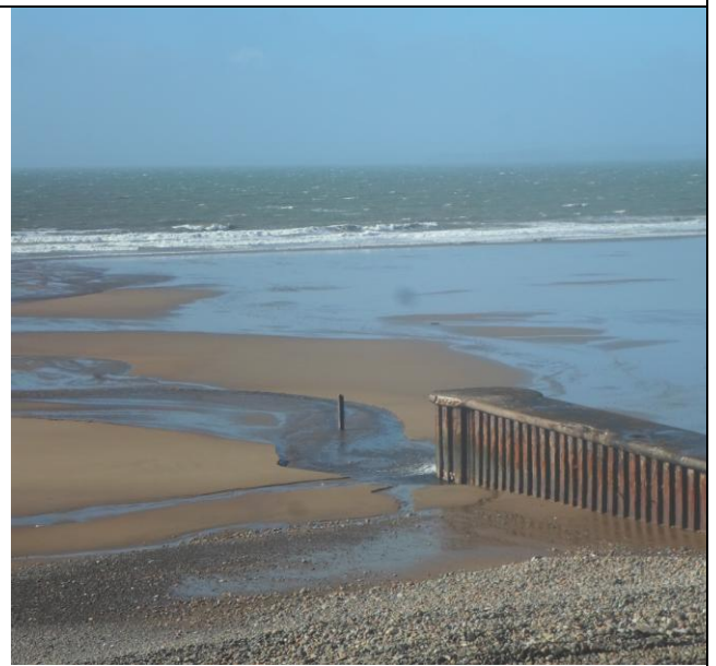
Photograph 8: Abbey beach outfall for floodwater surface drainage to Swansea Bay.
