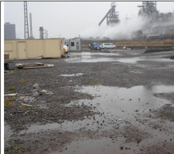
Photograph 1: Drainage on site
