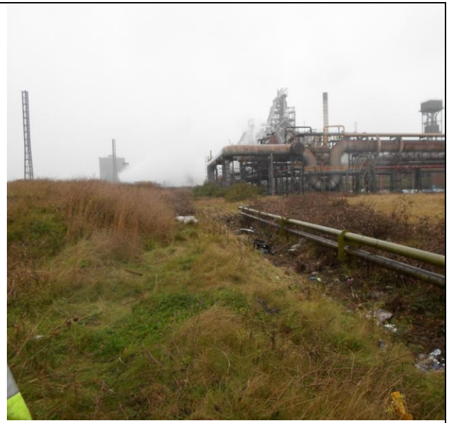
Photograph 2: Ditch with pipe running through
