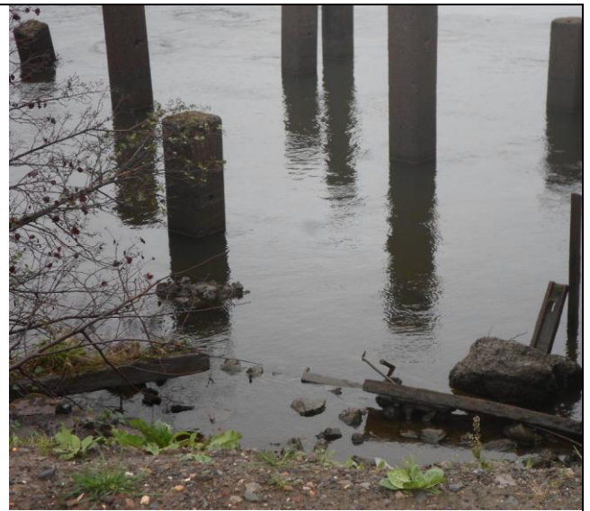
Photograph 6: Port Talbot Dock abstraction point for current cooling towers
