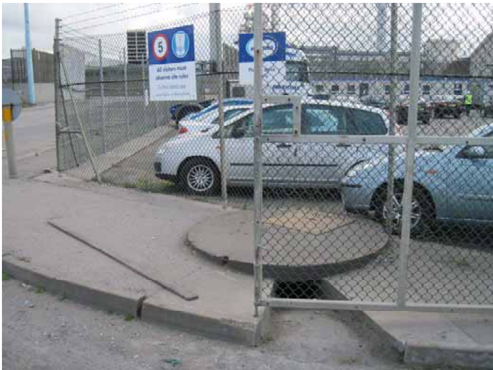
Maritime Entrance (Surface Drainage)
