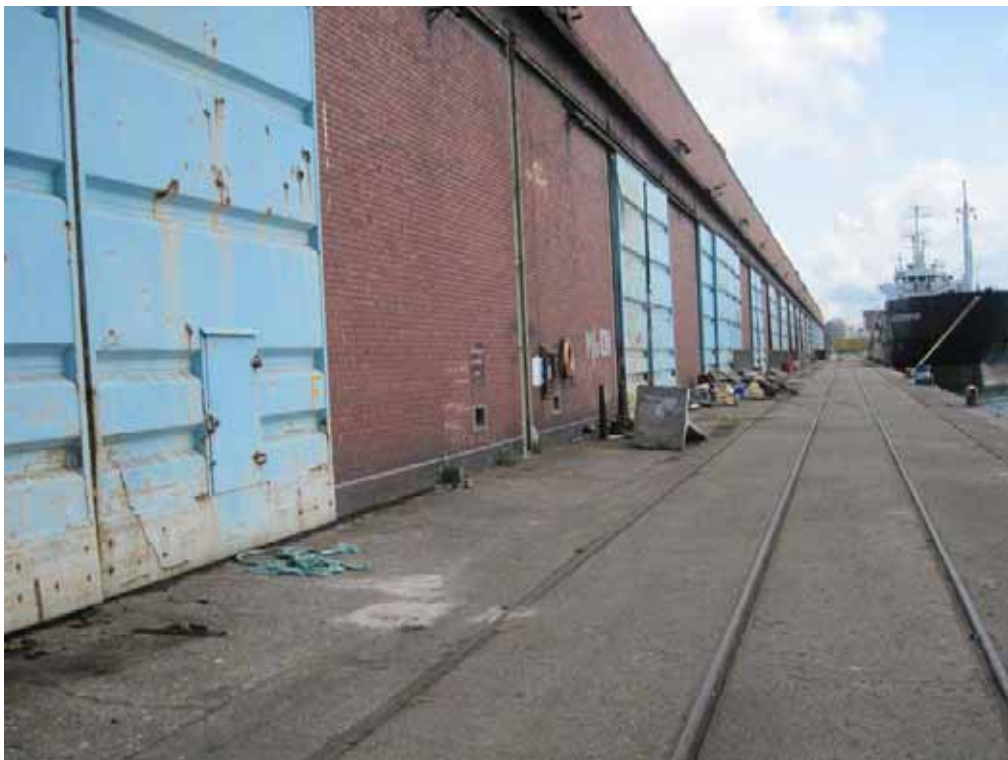
Alexandra West Shed
