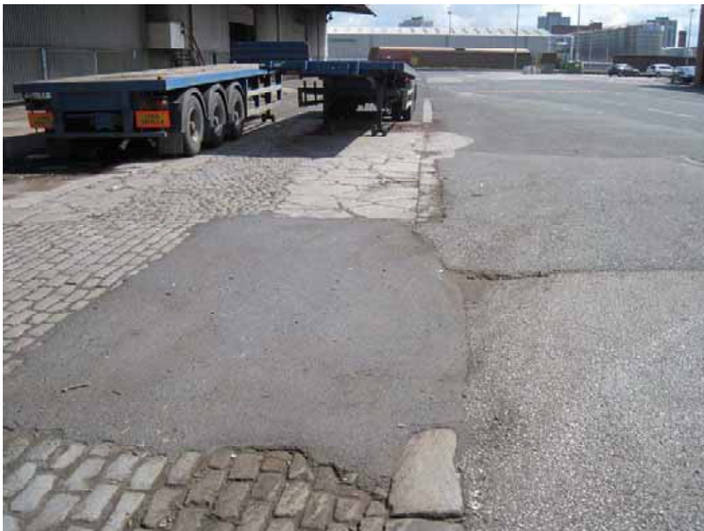
Road Surface Between Alexandra & Hornby Sheds
