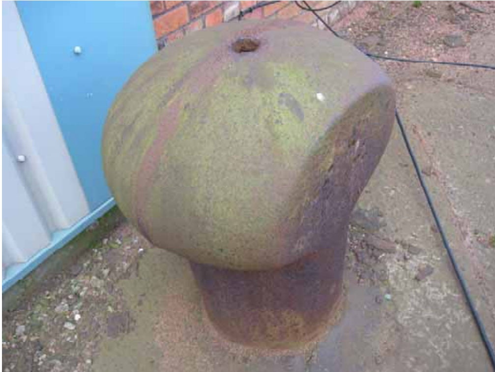
Disused Bollard Adjacent to Rock Bund
