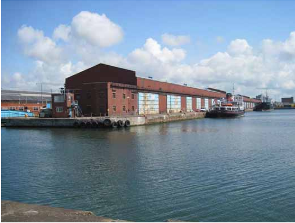
Alexandra Quay West Shed
