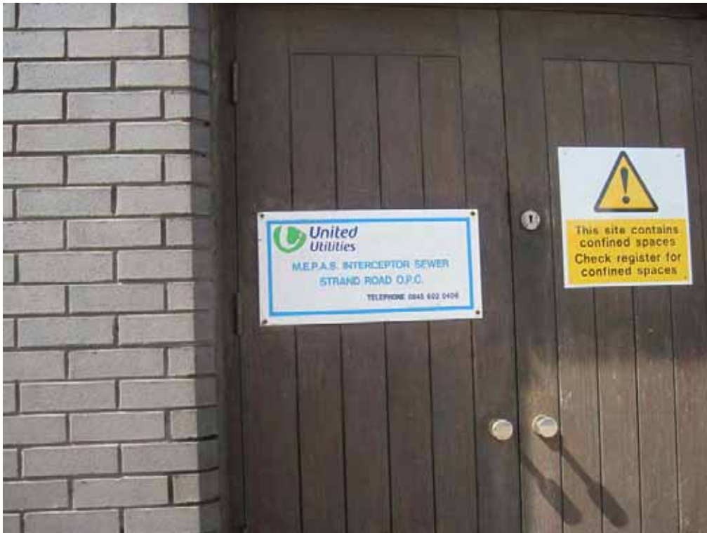
River Wall Interceptor
