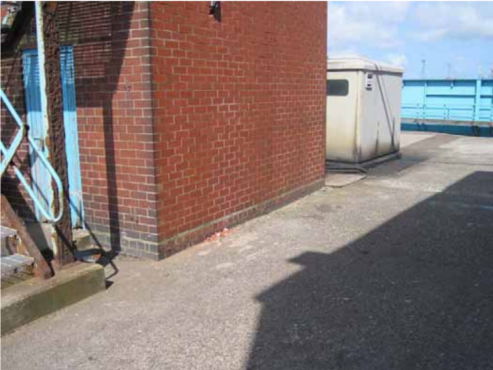
Canada 90' Swing Bridge Hydraulic Controls
