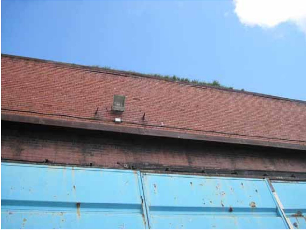
Alexandra West Shed
