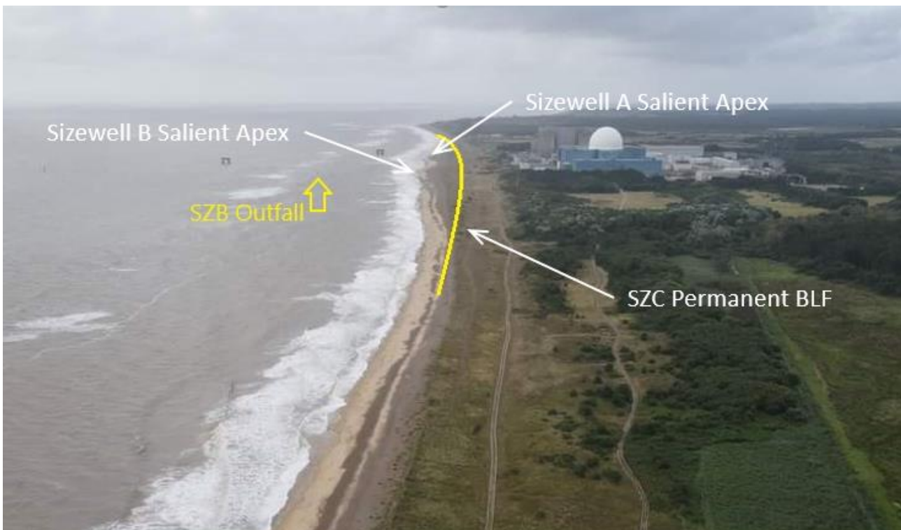
Figure 3: Embayed line for Sizewell Bay and SZC ZOI with BLF and SZA & SZB Salient
