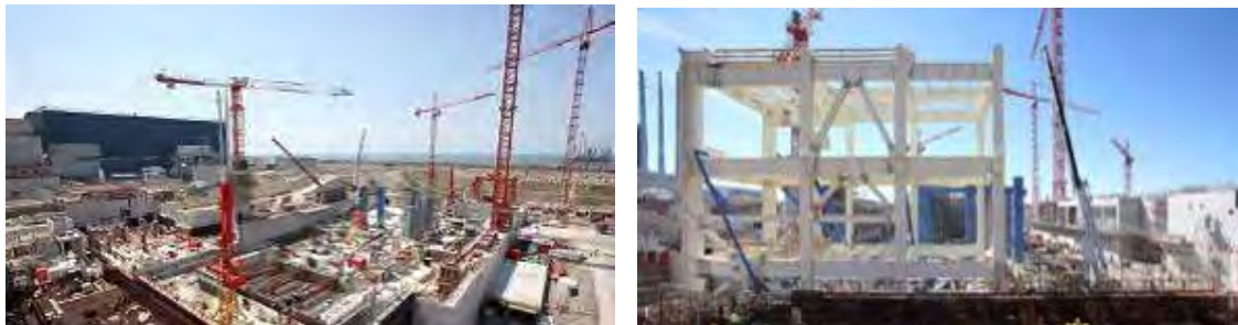
Figure 4.3: Construction of Buildings (Flamanville 3 – France)
