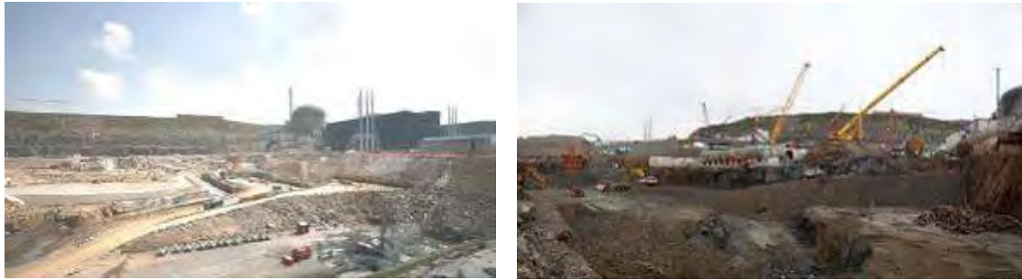
Figure 4.2: Site Preparation Works (Flamanville 3 - France)
