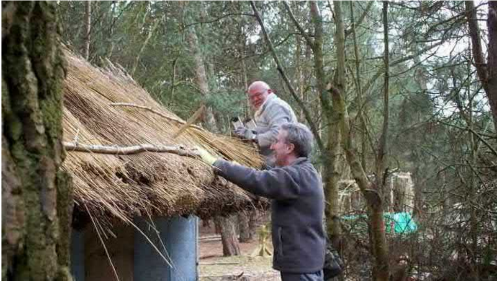
Sizewell reed being used to thatch an Iron Age dwelling at Iken (Photo: Duncan Allen)
