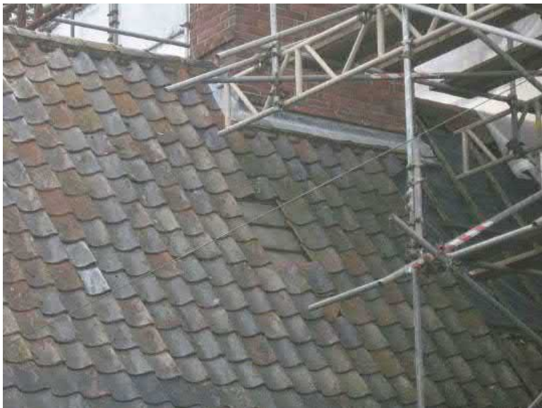
Photograph 2 Example of tiles missing from northern section roof
