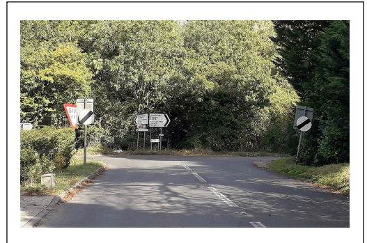
Photo 1 – View of the give way sign obscured by the speed limit signs
