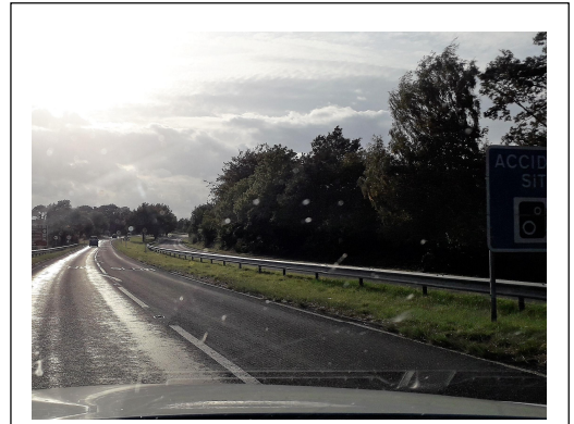
Photo 1 – View of A12 southbound approach to proposed roundabout
