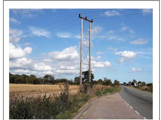
Photo 1 – Power line poles to the rear of the layby
