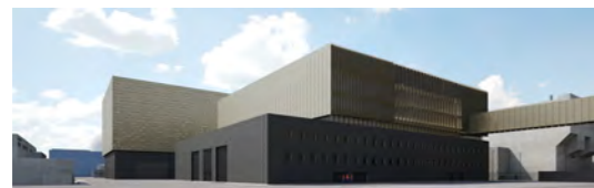
View of Eastern Elevation to the Operational Service Centre within the context of the Turbine Halls
