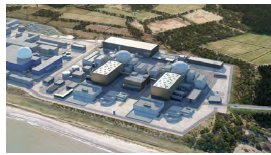
Aerial view of Sizewell C Operational Site
