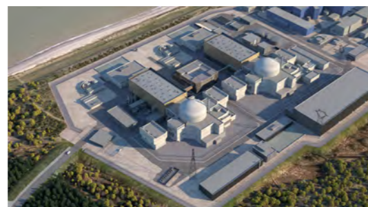
UK EPR™ Safety Related Buildings aerial view
