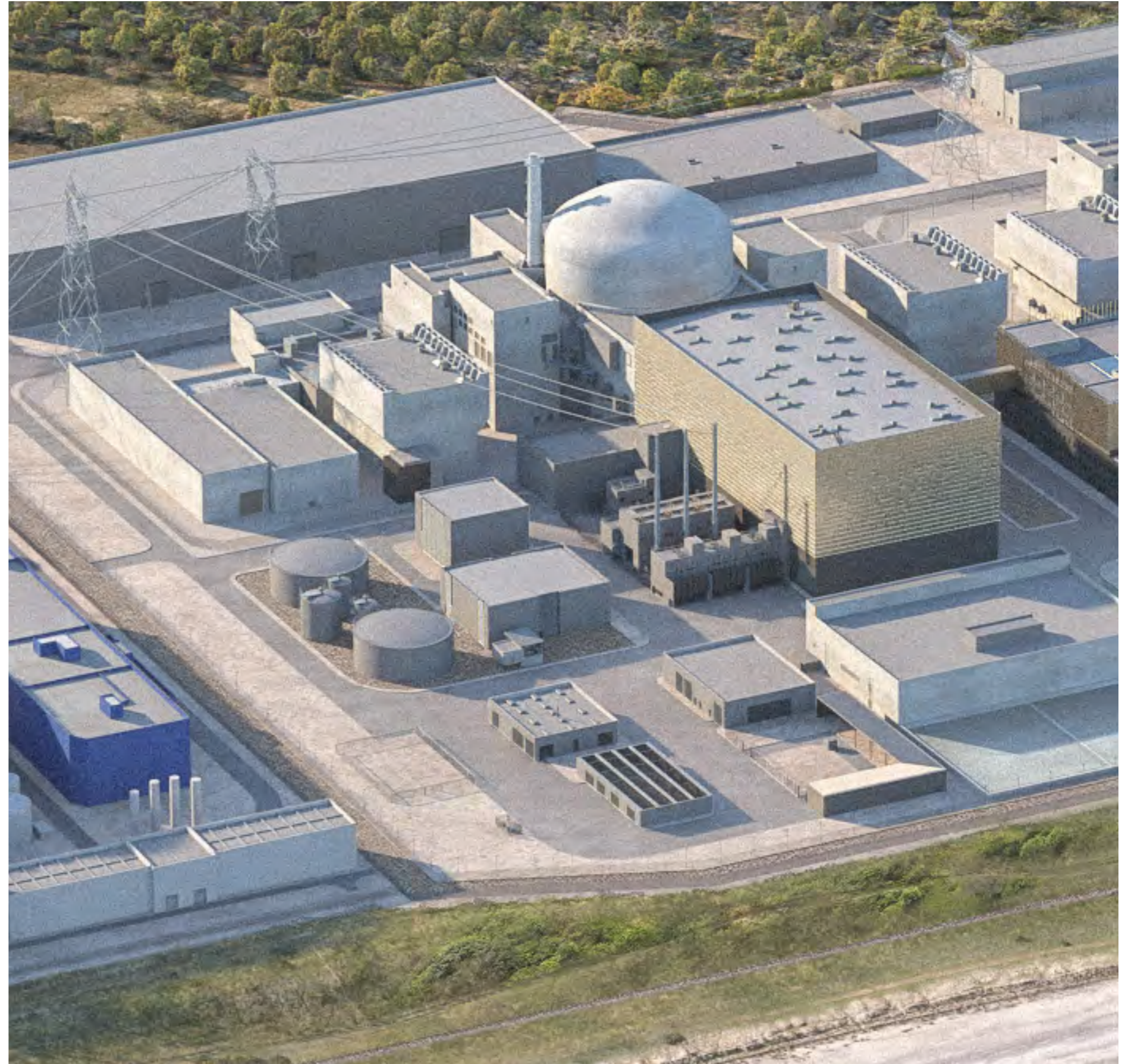
Figure 7.74: Ancillary buildings aerial overview including plant and storage facilities
