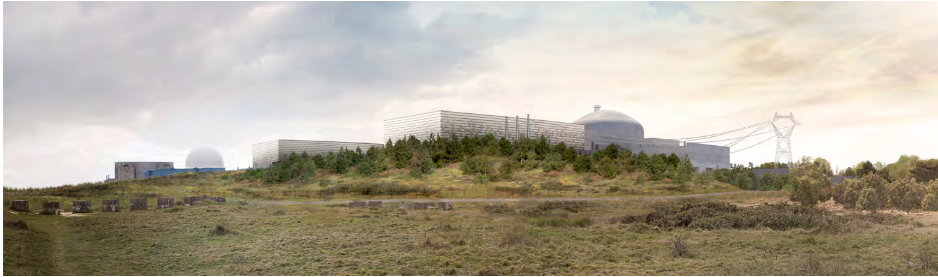
Figure 7.45: Light bronze facade treatment to the turbine halls of Sizewell C (refer to Figure 13.10.24 of Volume 2, Chapter 13 of the ES)
