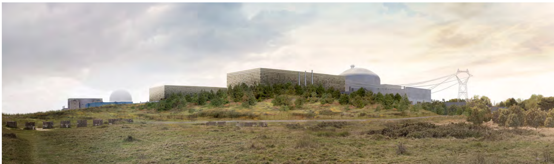
Figure 7.47: Darker bronze facade treatment to the turbine halls of Sizewell C (refer to Figure 13.10.24 of Volume 2, Chapter 13 of the ES)
