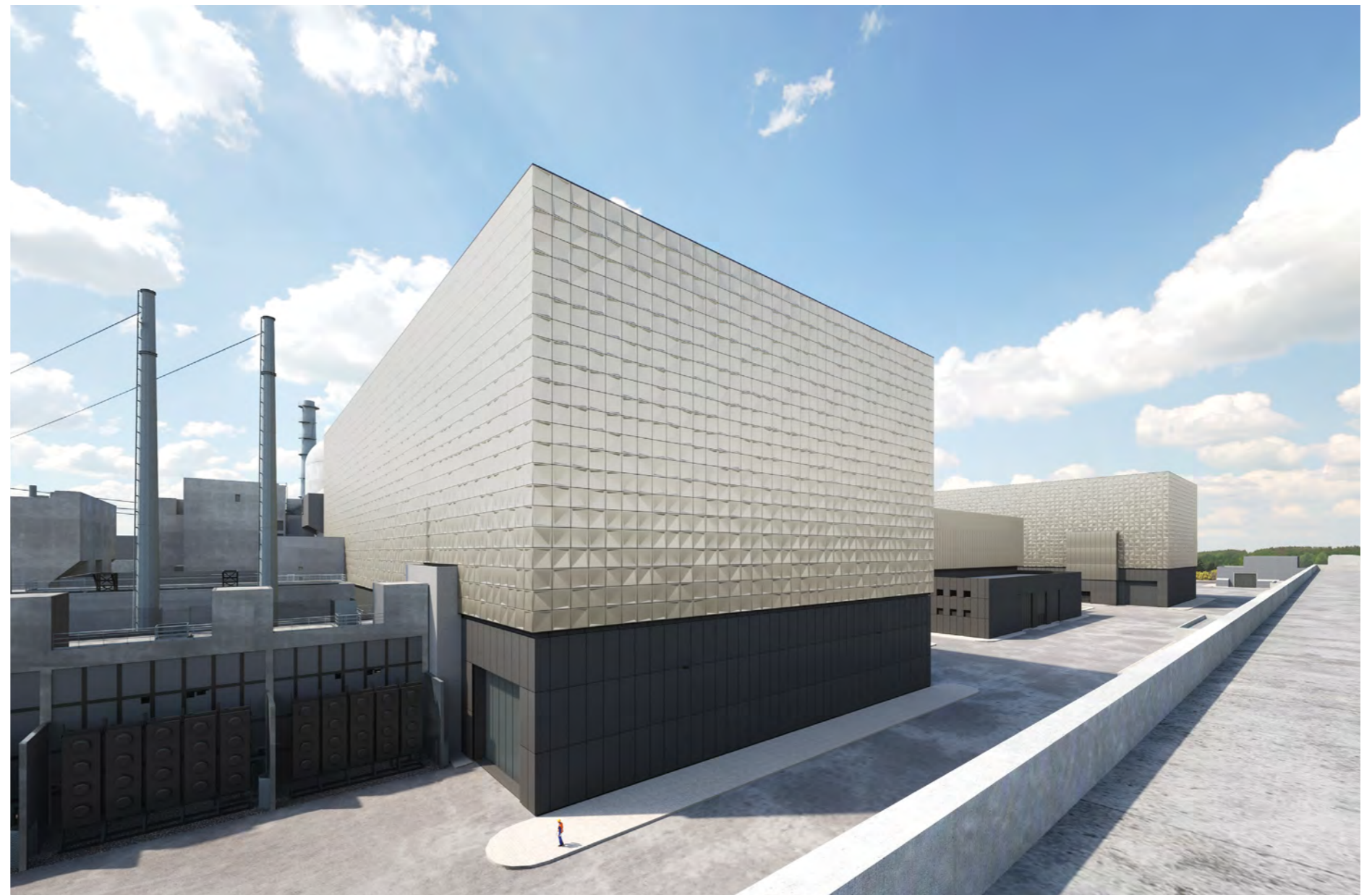
Figure 7.59: View showing the eastern elevation and building sequence of the operational service centre between the turbine halls
