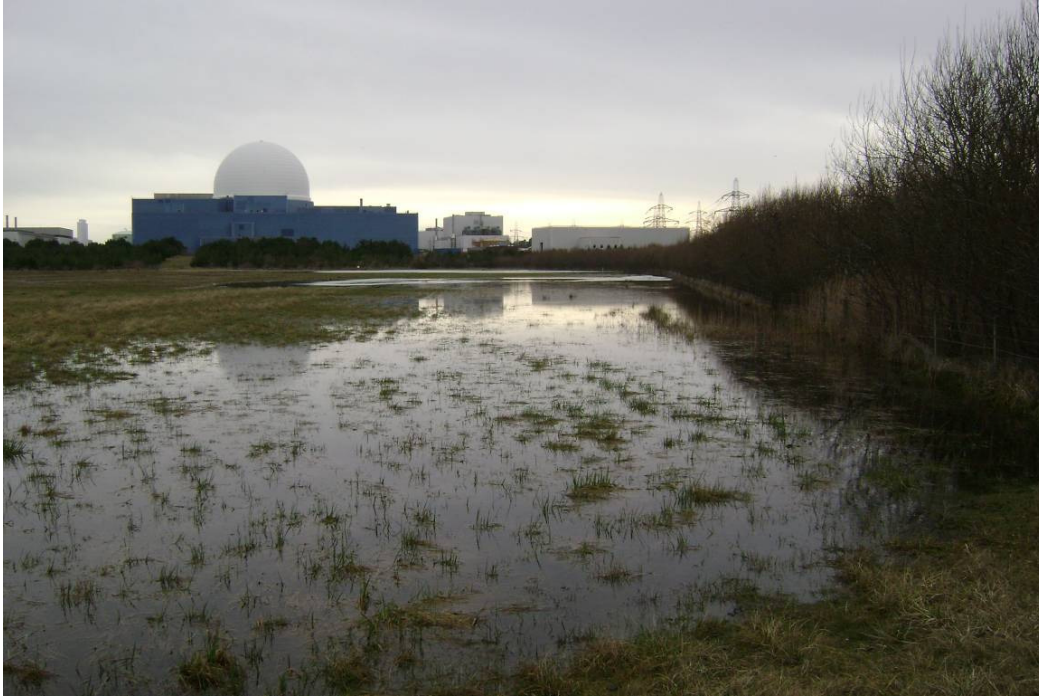
Figure 4: Example of inaccessible location – waterlogged ground
