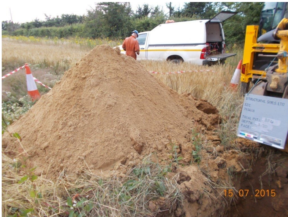
TP BP3 - SPOIL
