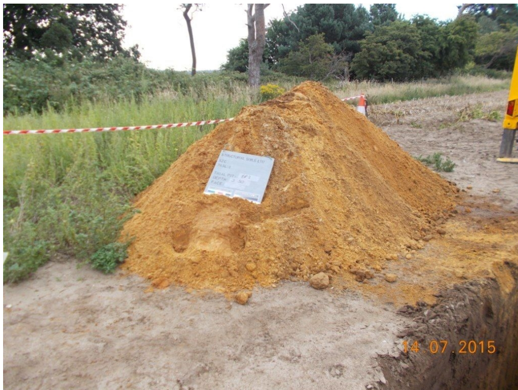
TP BP2 - SPOIL
