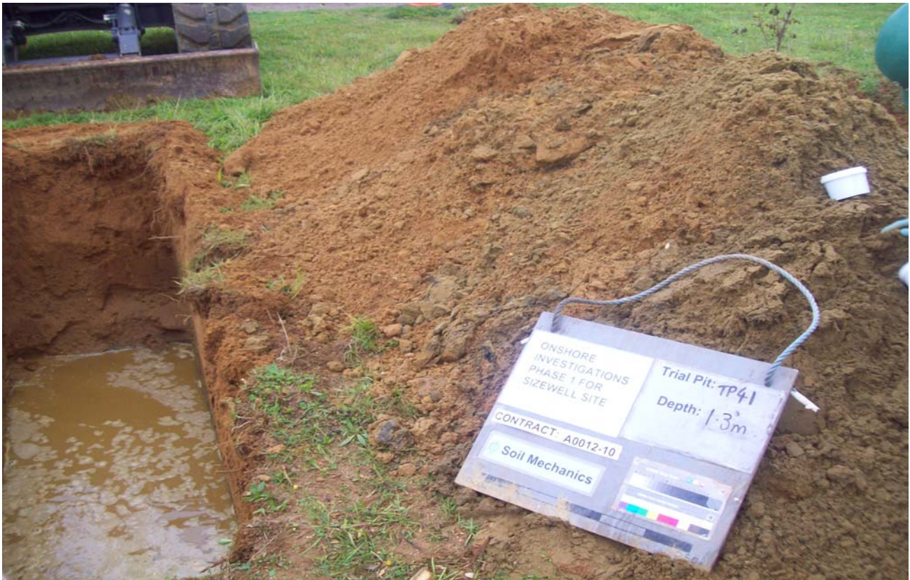
Trial Pit 41 Spoil
