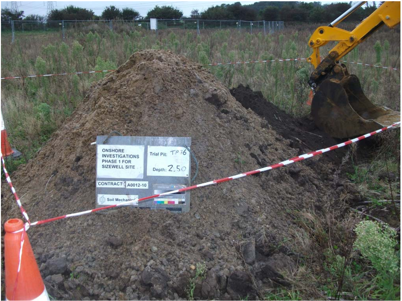
Trial Pit 76 Spoil
