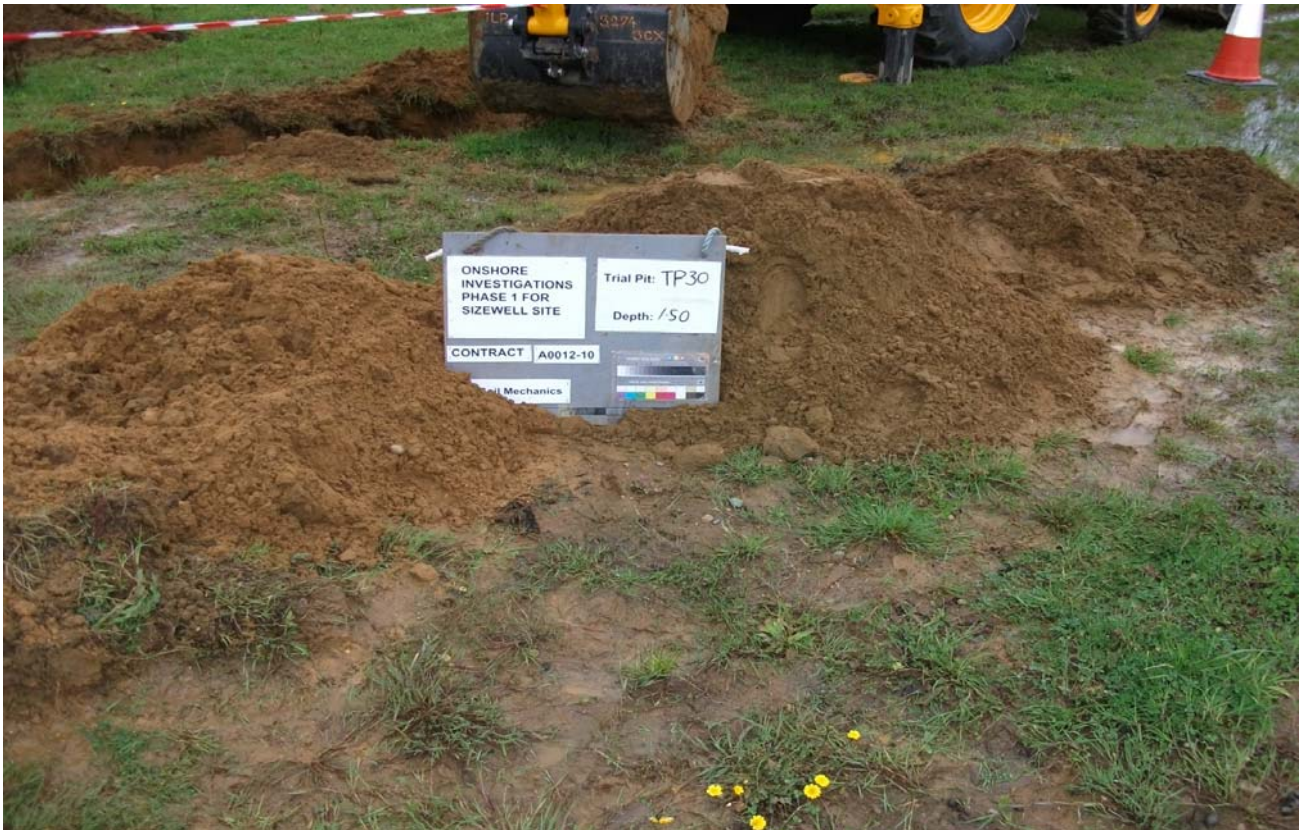
Trial Pit 30 Spoil
