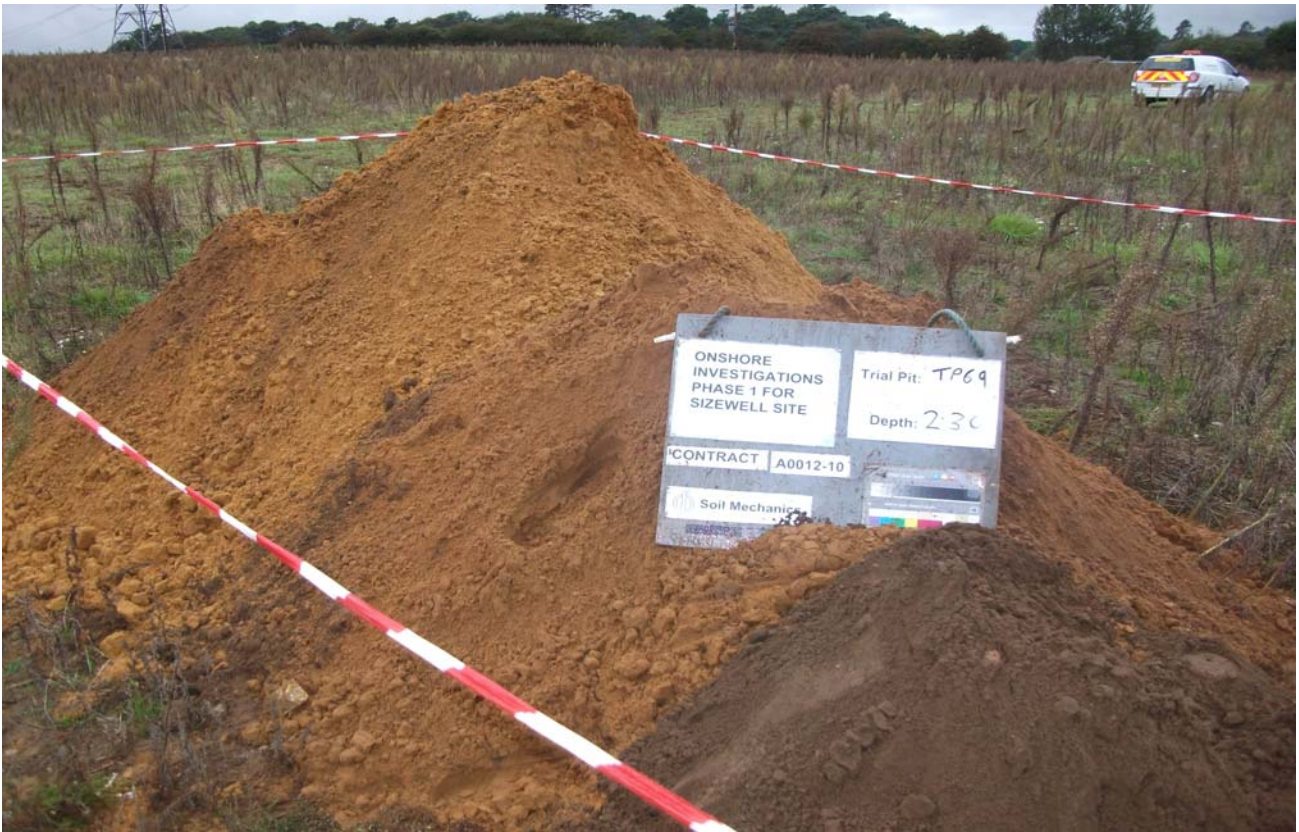
Trial Pit 69 Spoil
