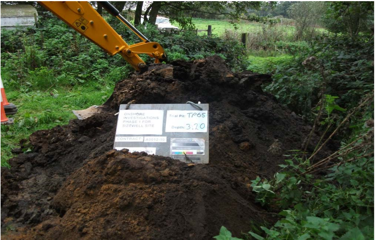
Trial Pit 65 Spoil
