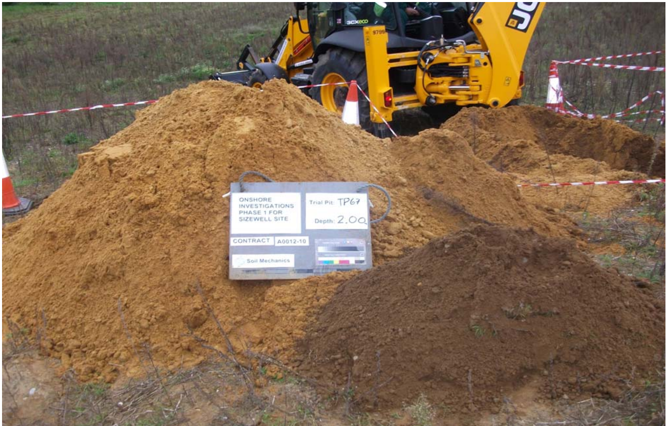
Trial Pit 67 Spoil
