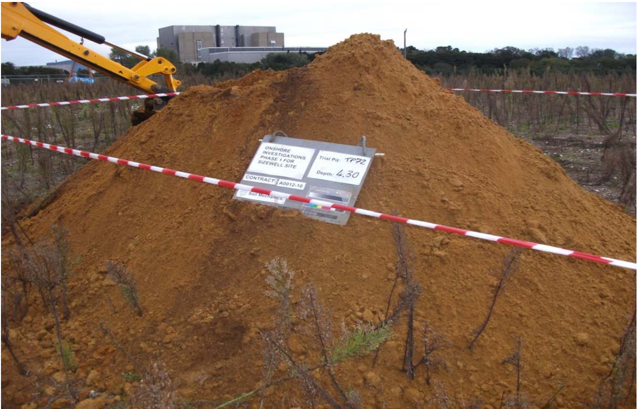
Trial Pit 72 Spoil
