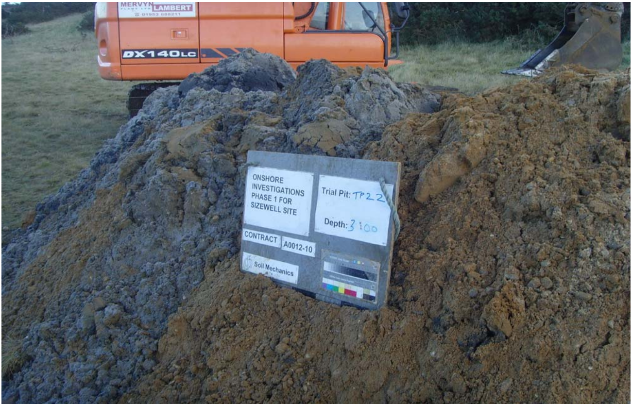
Trial Pit 22 Spoil
