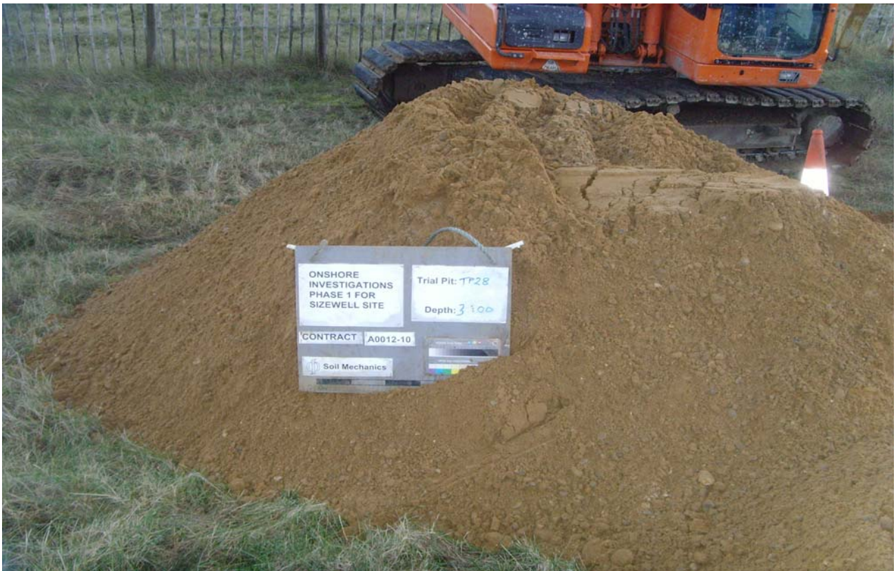
Trial Pit 28 Spoil
