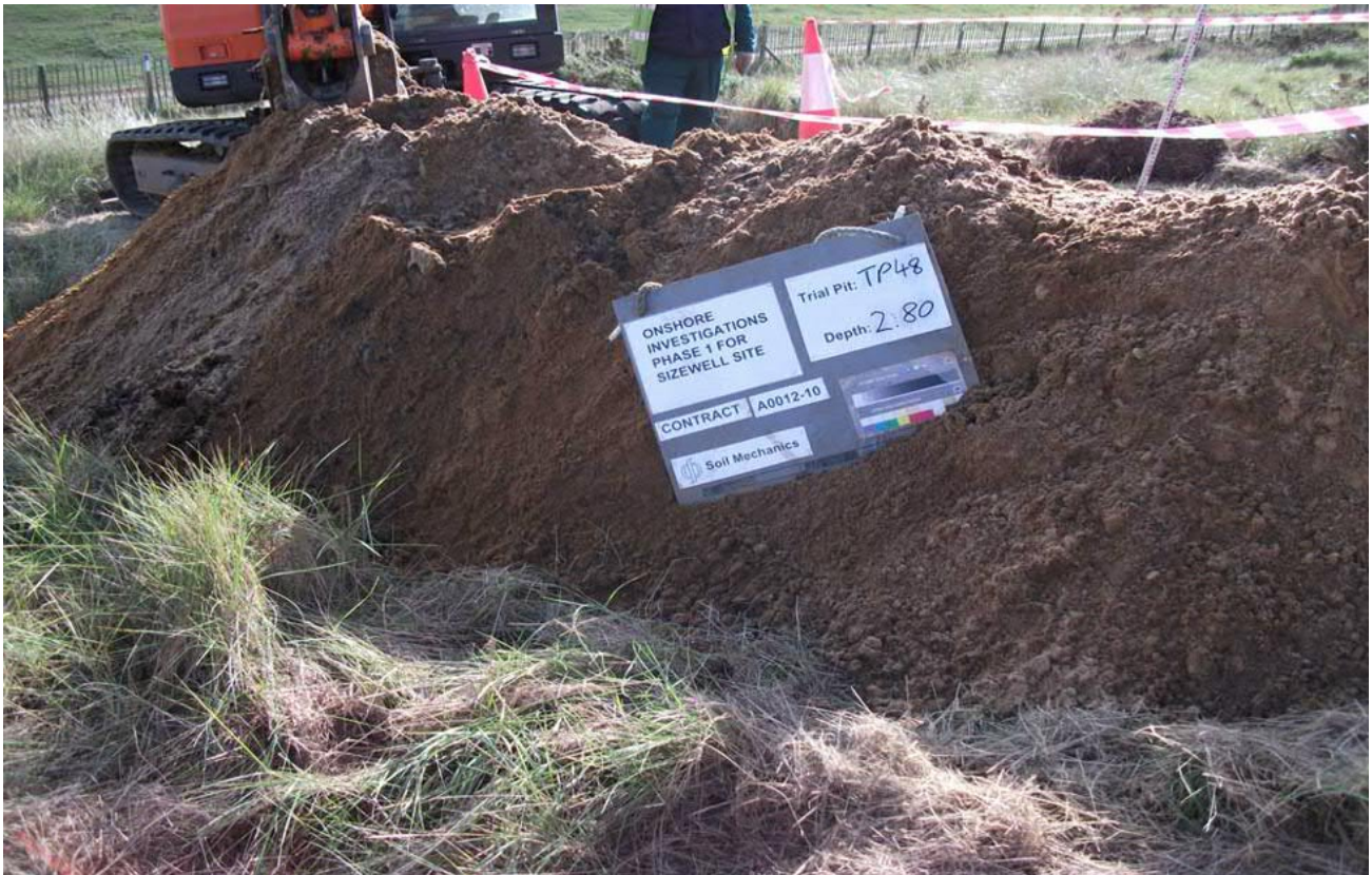
Trial Pit 48 Spoil
