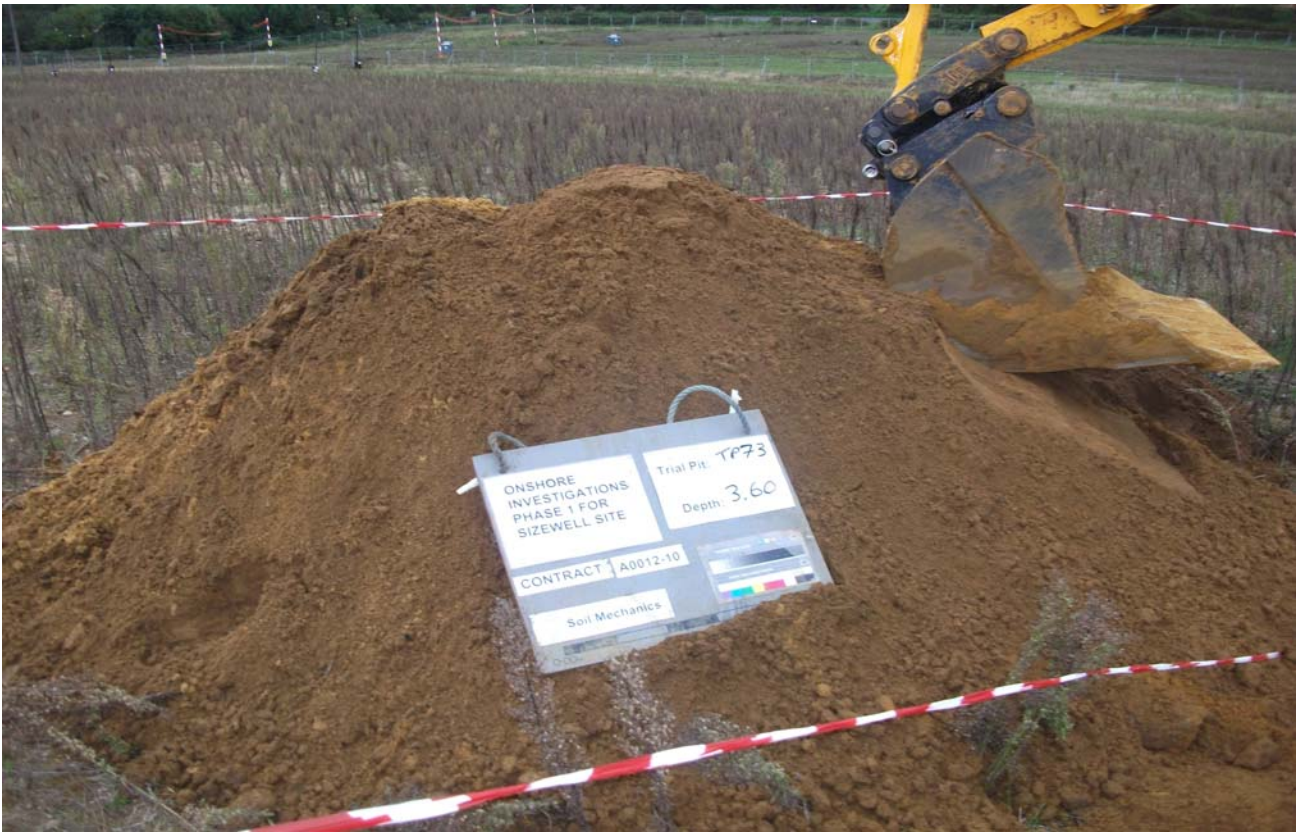
Trial Pit 73 Spoil
