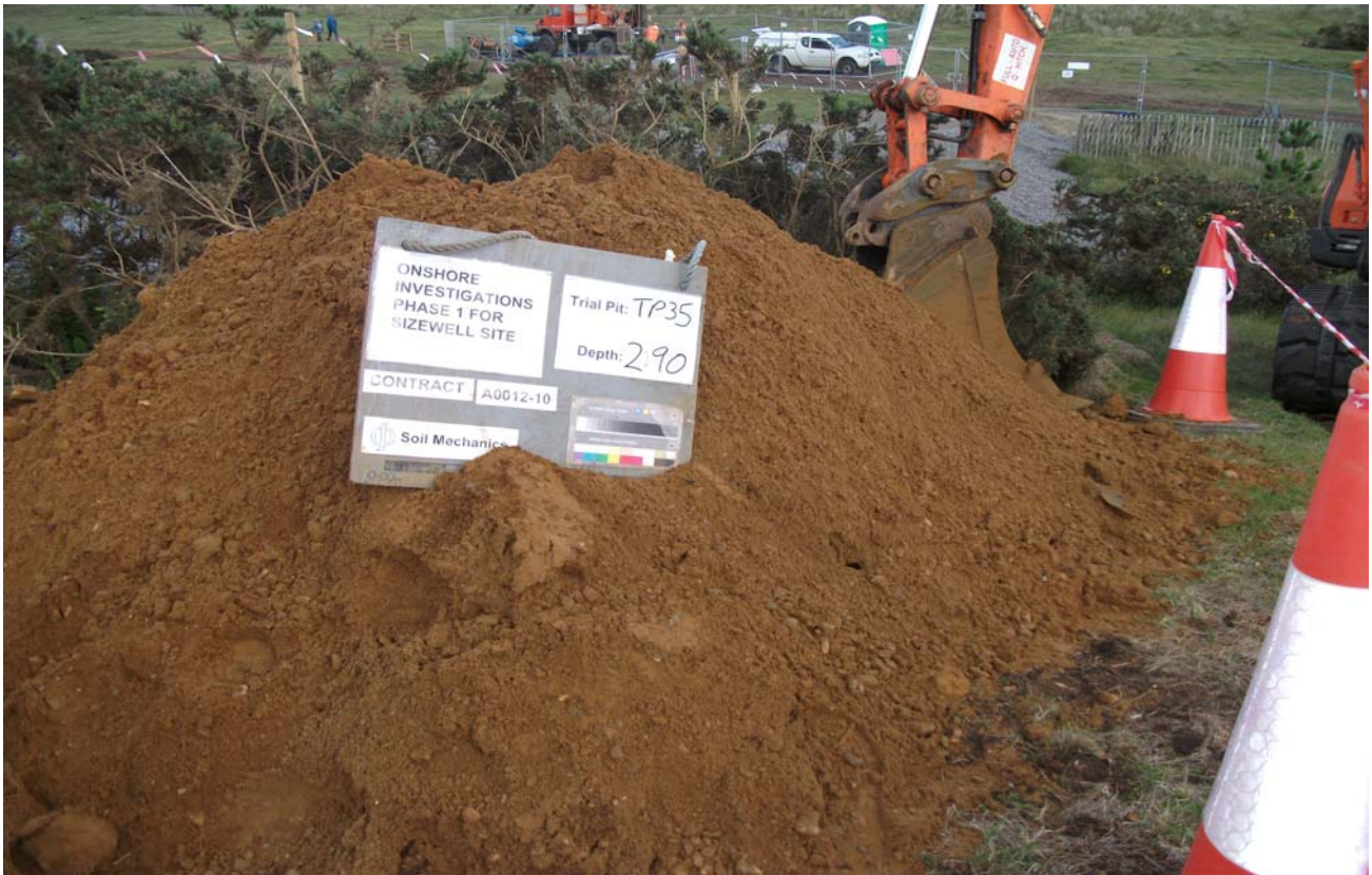
Trial Pit 35 Spoil
