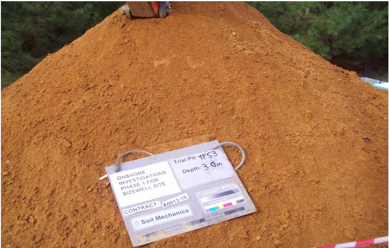
Trial Pit 53 Spoil
