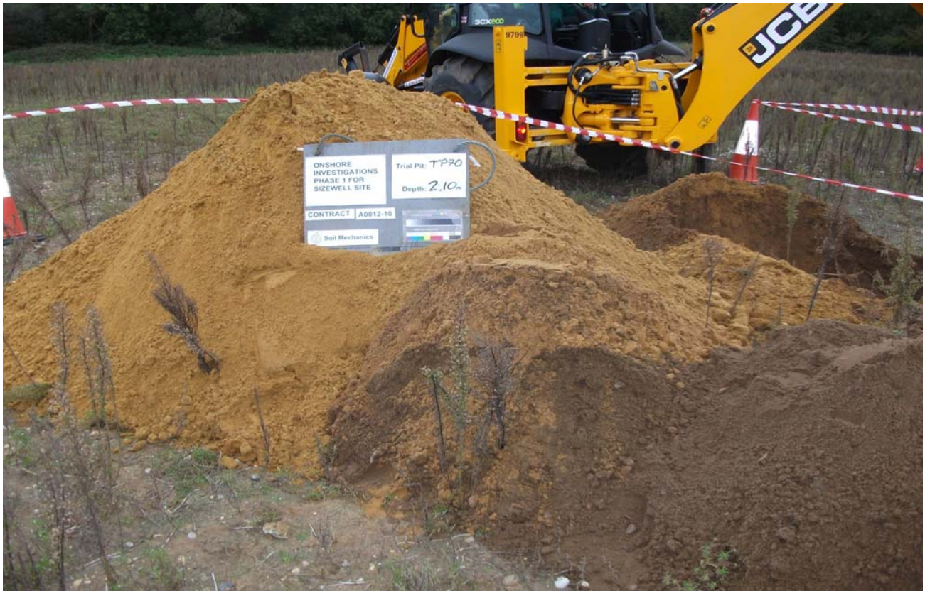
Trial Pit 70 Spoil
