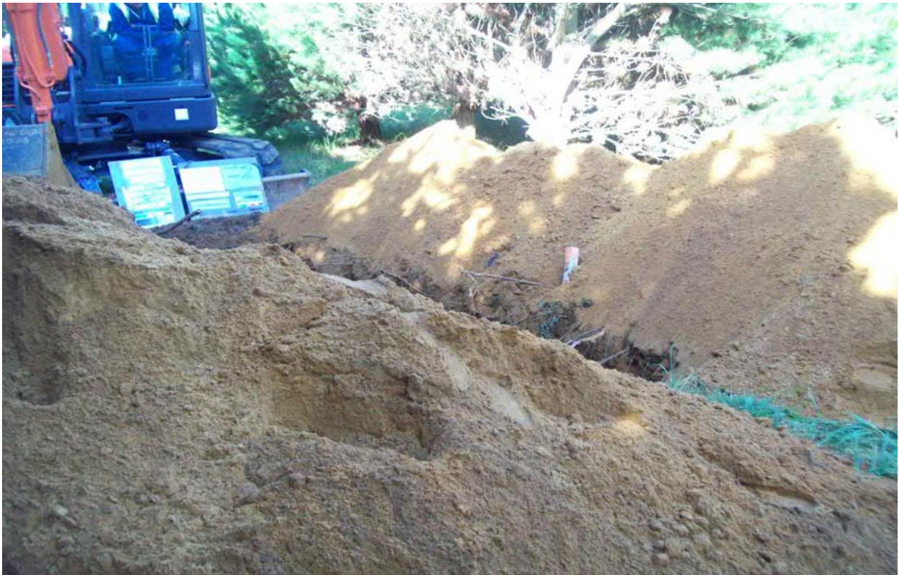
Trial Pit 52 Spoil
