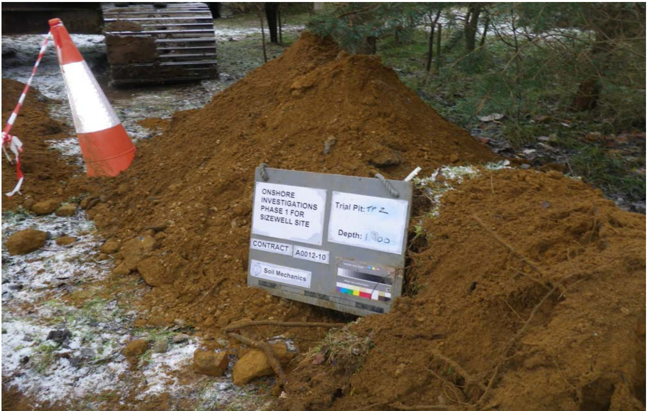
Trial Pit 2 Spoil
