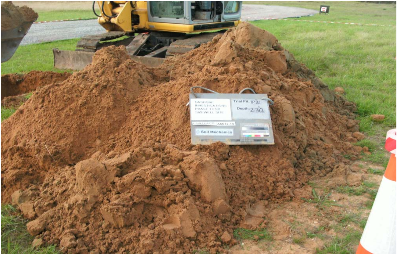
Trial Pit 21 Spoil
