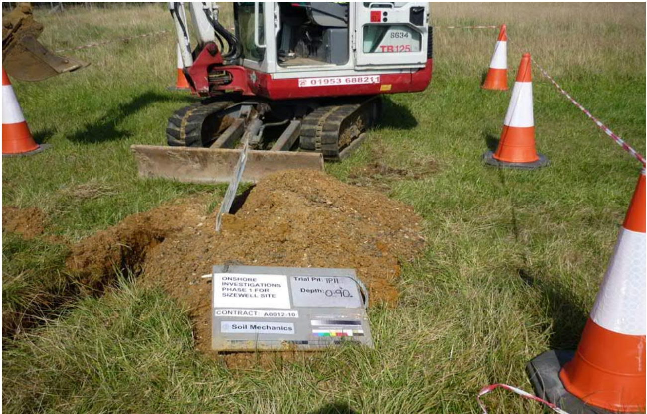
Trial Pit 11 Spoil
