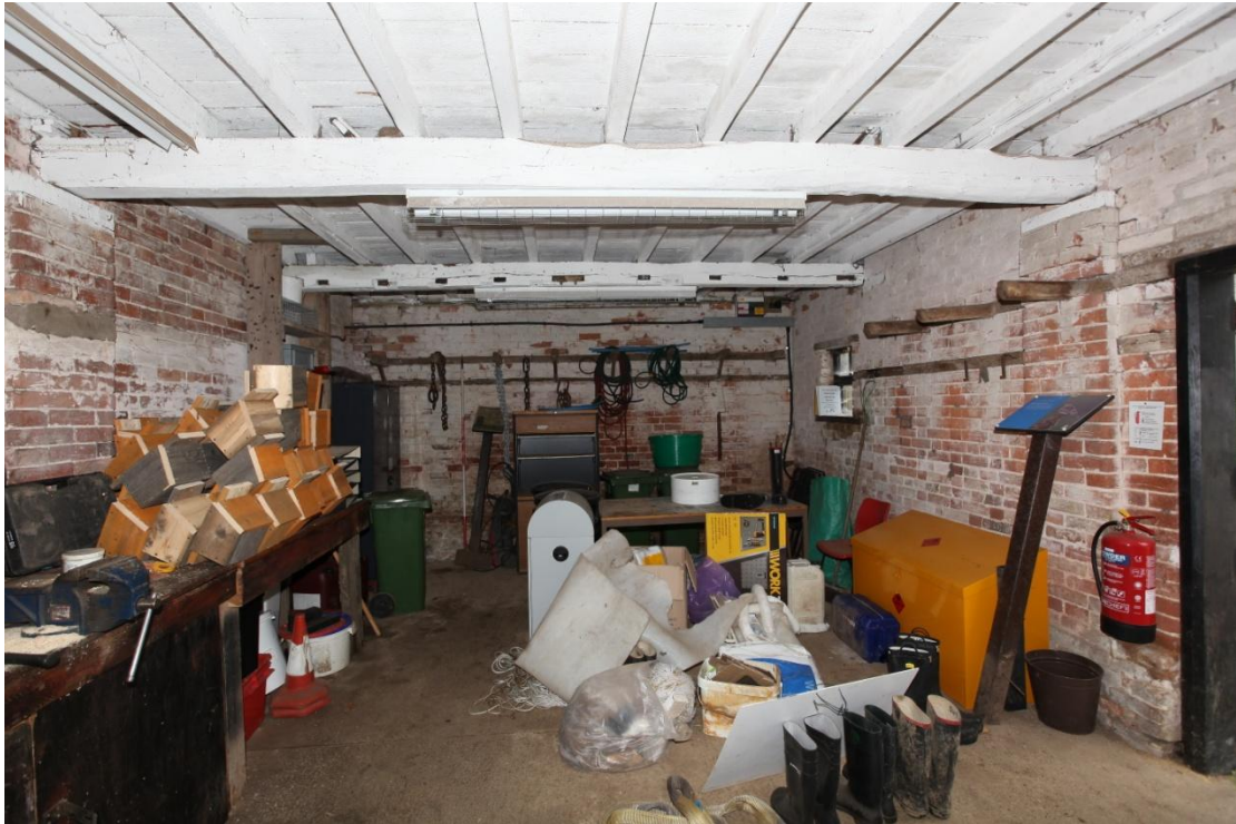
Illus. 17. The northern section of the stable (2b) as seen from the south showing a good series of original wooden harness hooks lining the walls with a blocked hay drop to the left. The floorboards above this drop are short insertions that are aligned differently to the boards elsewhere in the ceiling. The hay racks and mangers have been removed. The bind joist in the rear is a re-used timber with irrelevant empty mortices.
