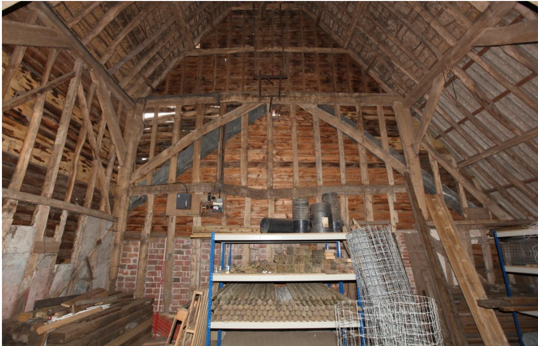
Illus. 11. The barn's symmetrical western internal gable (1) with a waney mid-rail, trenched braces and chiselled carpenter's numerals. This contrasts with the eastern gable where the mid-rail is interrupted by an additional post to the rear of its centre. The corner post on the left contains pegged mortices for an identical aisle tie-beam and brace to those on the right.
