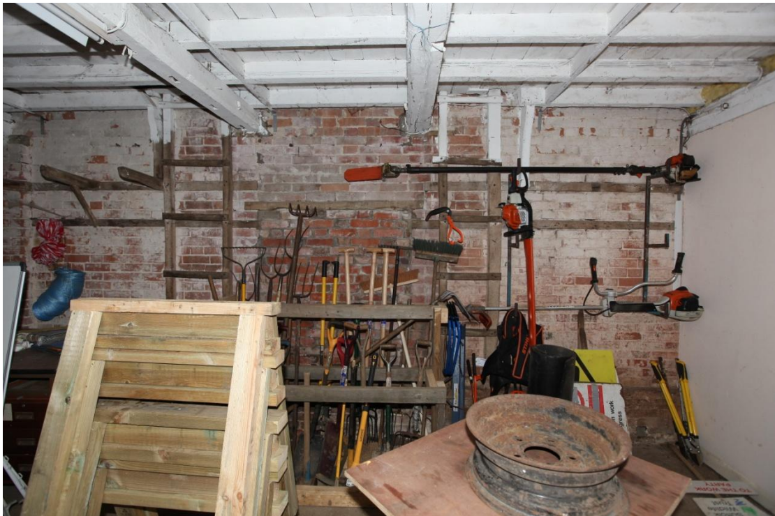
Illus. 16. The eastern interior of the stable's northern section (1b) showing the blocked central door between the two ostensibly original loft ladders with original wooden harness hooks on the left (and wooden rails set into the brickwork for others on the right). The principal joist to the left of the door contains empty mortices for a missing partition but there is no counterpart to the right.
