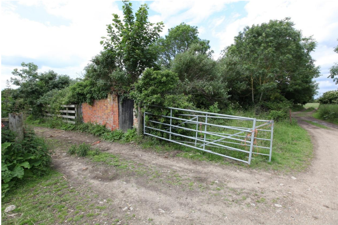
Illus. 23. The largely collapsed northern cattle shed viewed from the south-east (6) with its dated plaque to the left. Fragments of a flint-rubble eastern wall with red-brick dressing are hidden in the undergrowth and the doorway to the right of the scale rod is an original feature respected by closers – as is the former gateway on the left.
