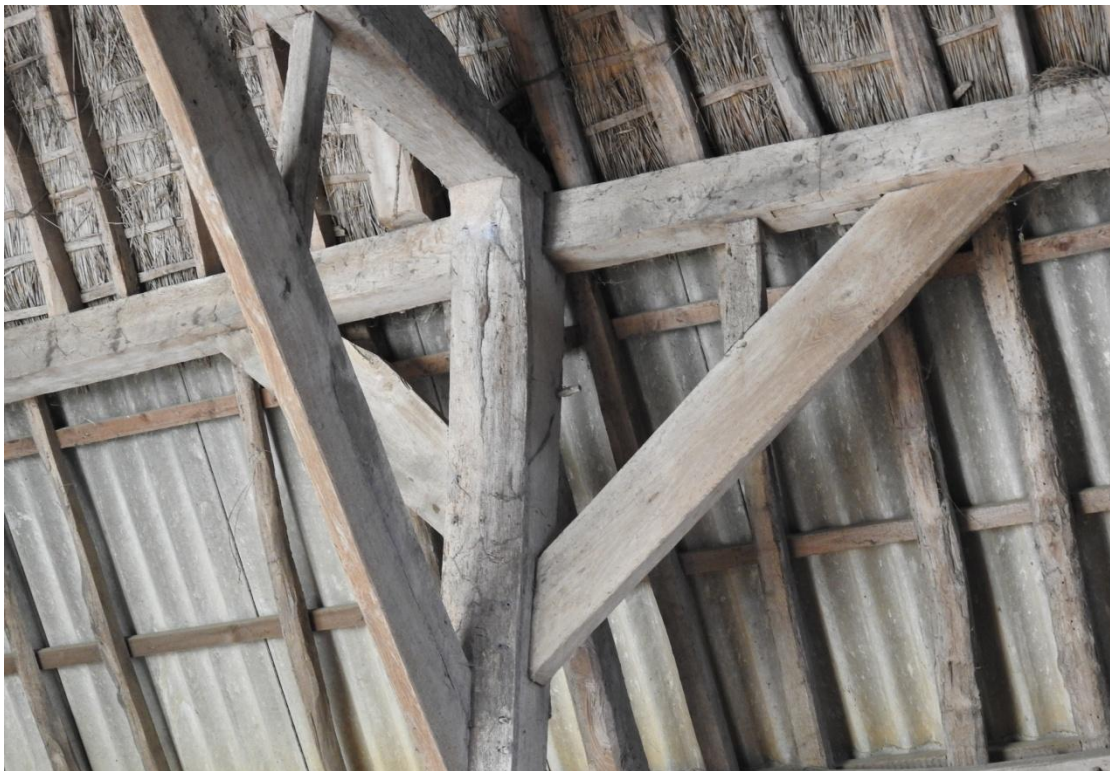
Illus. 8. The arcade post to the right of the easternmost entrance showing its exceptional spandrel struts and the smaller arcade brace to the threshing bay. Every tie-beam brace contains identical struts but the barn contains only two arcade-brace struts – both beneath scarf joints and both flanking a threshing bay. The struts are re-used timbers.
