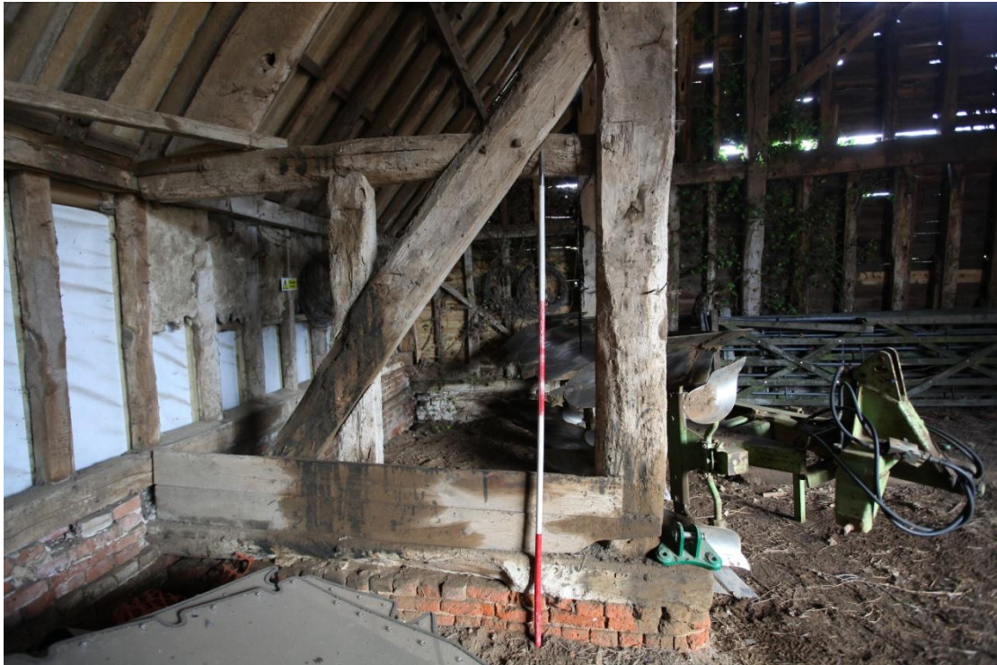
Illus. 9. The easternmost truss of the barn's aisle (1) as seen from the west. The single, large stud and thick, slightly waney aisle brace and tie-beam with hewn surfaces are typical of the Middle Ages and contrast with the sharp-edged, uniform timber of the upper braces and other key elements such as the arcade-plates. A truncated mortice for a jowled wall post in the left-hand end of the aisle tie proves that the wall framing has been rebuilt or the timbers have been re-used – or both.
