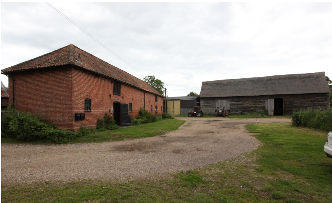
Illus. 2. The main yard from the south showing the brick stable (2) and the thatched and weatherboarded barn (1). Note the asymmetry of the barn's facade, with one of its two sets of entrance doors in the second bay from the left and the other in the third bay from the right. Although of traditional braced construction both doors are in excellent condition and appear to be 20 th century replacements. The steel-framed shed to its left is modern.
