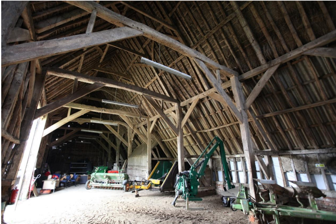
Illus. 5. A general view of the barn's interior from its south-eastern corner (1). All seven bays are visible along with the floor of loose earth with no trace of the threshing floors onto which the two southern entrances would have opened. The rear aisle to the right was initially replicated on the left but the structure is otherwise exceptionally intact with only one missing tie-beam brace. The aisle is not a later addition as stated in the listing as there are no stud mortices for an earlier back wall in the arcade-plate.
