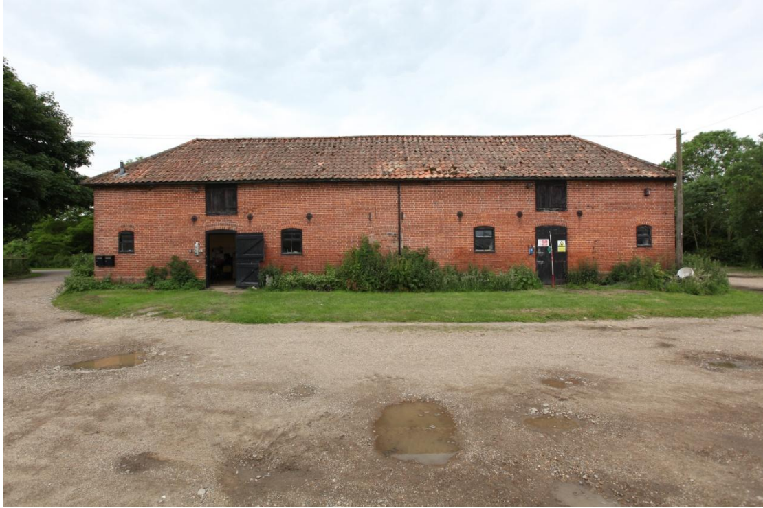
Illus. 15. The eastern facade of the pantiled brick stable (2) showing its symmetrical twin entrances, loft hatches and windows. The outline of a third blocked door is visible in the centre. This would normally have opened onto an internal loft stair, but there is no obvious evidence of this in the ceiling and it probably served a tack room.
