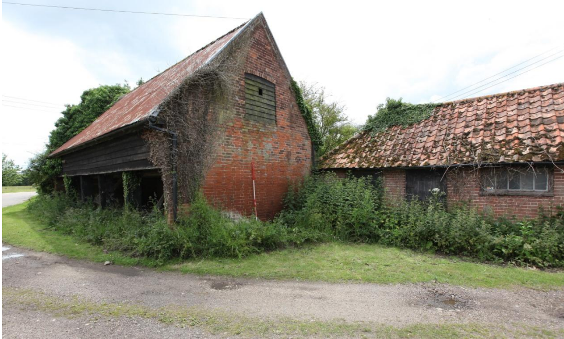
Illus. 19. The cart lodge (3) from the north-east showing the blocked granary loading hatch or louver in its gable with the small cart shed and stable (4) on the right. Four sets of initials lie at vertical intervals to the right of the scale rod, three of which are dated 1797.
