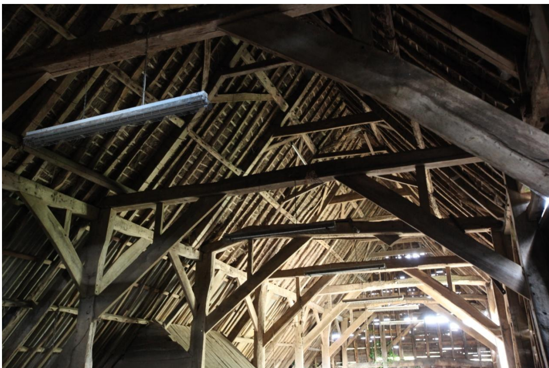
Illus. 6. A general view of the barn's impressive roof (1) from the west showing its complete array of tie-beam and arcade-plate braces with a full complement of wind-braces in the two-tier roof of linear butt-purlins.
