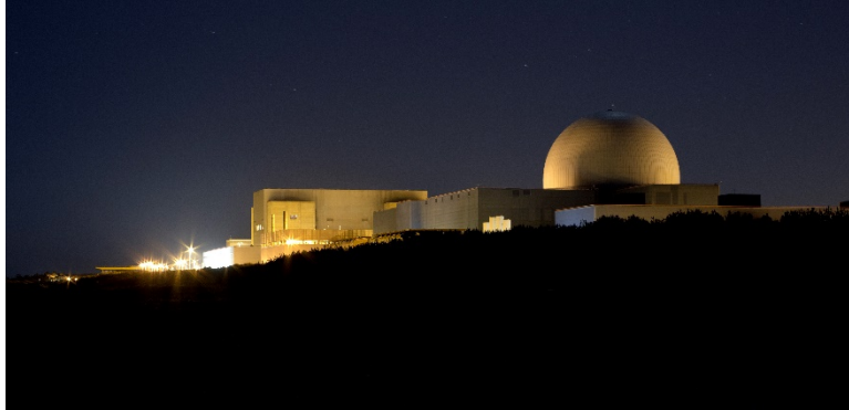
Plate 1.3: Typical view of existing lighting at Sizewell A & B Power stations
