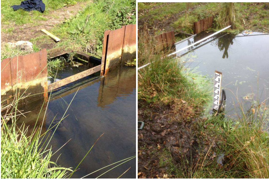
Figure 6: Photos of Site 4, pre and post weir plate movement.
