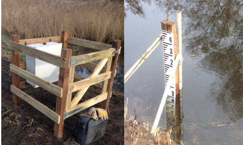
Figure 1: Enclosed Cabinet and Gaugeboard installation (Site 1)
