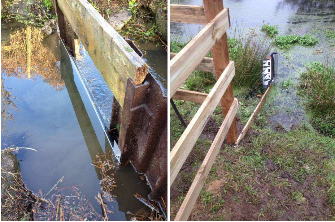
Figure 5: Photos of Site 3 installation
