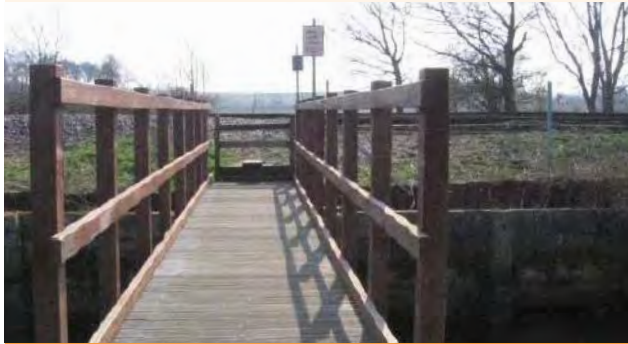
Figure 9.18 Current Melton Bromswell level crossing (ID SWC27)
