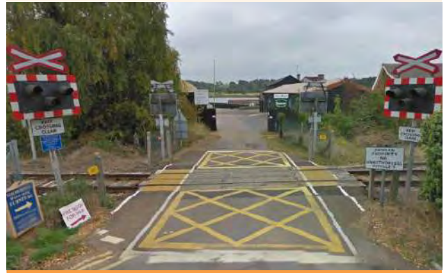
Figure 9.46 Current Sun Wharf level crossing (ID SWC18)
