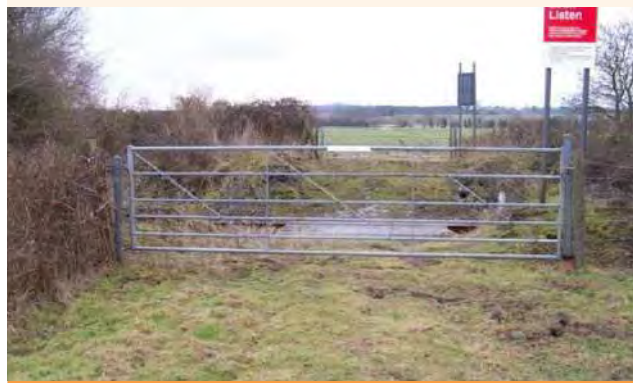
Figure 9.87 Current Snowdens level crossing (ID SWC51)
