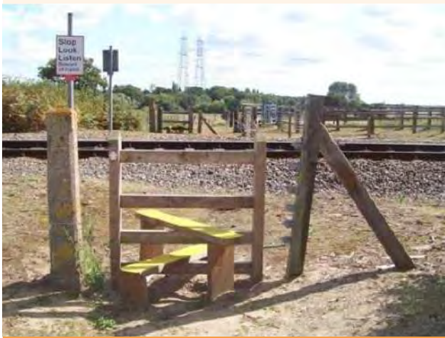
Figure 9.72 Current Farnham level crossing (ID SWC41)
