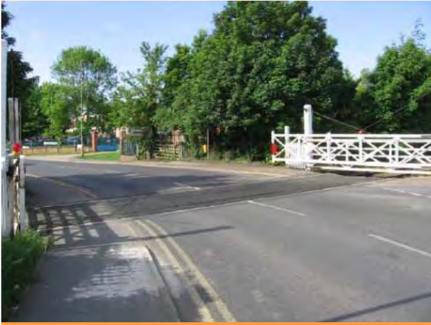
Figure 9.82 Current Leiston level crossing (ID SWC55)
