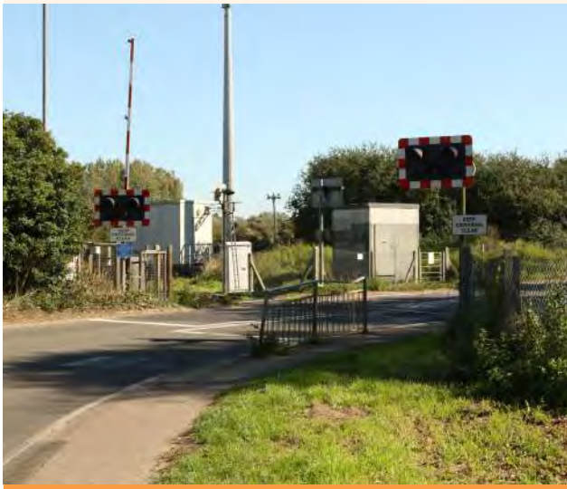
Figure 9.48 Current Melton Station crossing (ID SWC24)
