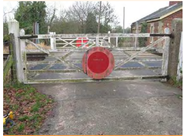
Figure 9.74 Current Brick Kiln level crossing
