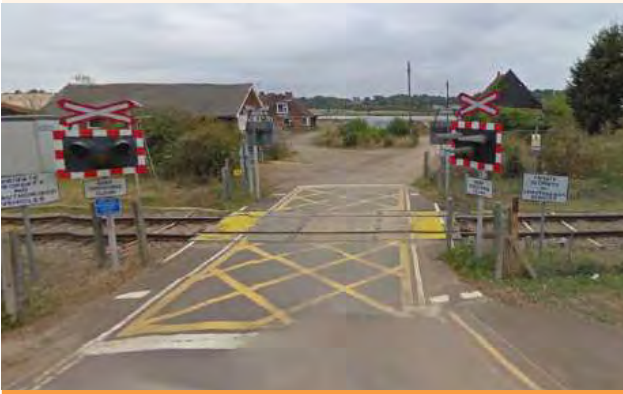
Figure 9.45 Current Lime Kiln Quay level crossing (ID SWC17)
