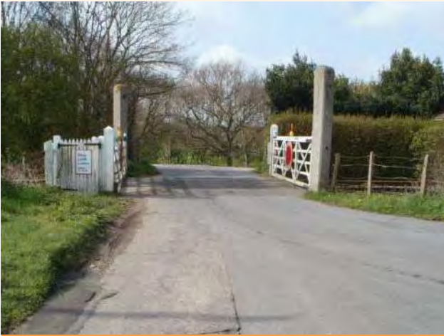
Figure 9.80 Current Saxmundham Road level crossing (ID SWC52)
