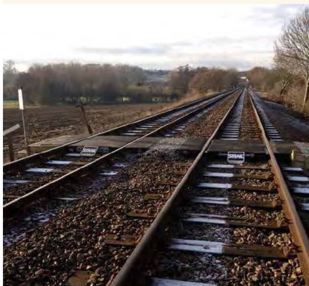
Figure 9.15 Current Martlesham level crossing (ID SWC09)
