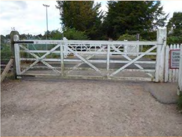
Figure 9.59 Current Jetty Avenue level crossing (ID SWC13&14)
