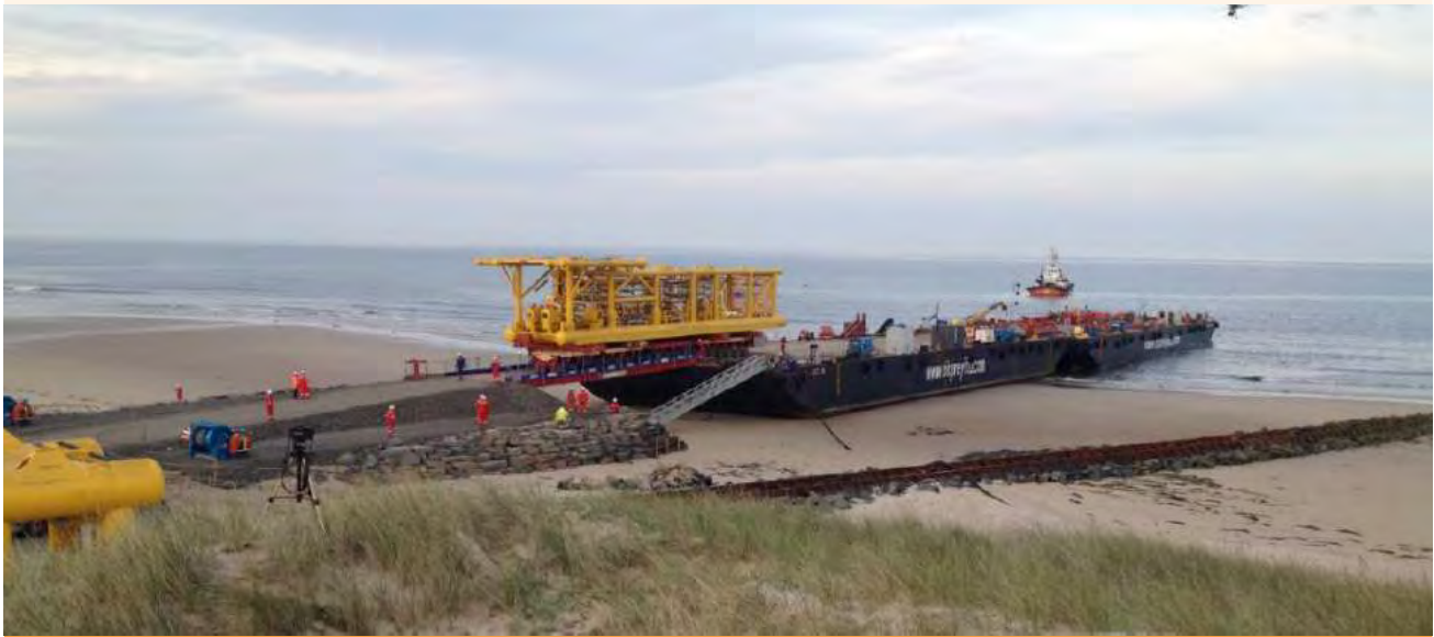
Figure 7.51 Example of a Beach Landing Facility
