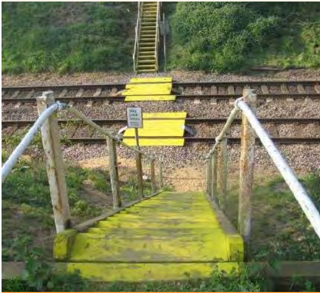
Figure 9.5 Current Lacy's footpath level crossing (ID SWC03)
