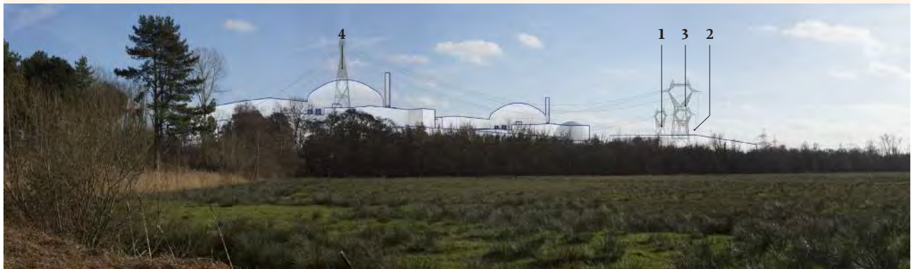
Figure 7.11 National Grid connection, view looking south-east from Sandlings Walk at Goose Hill
