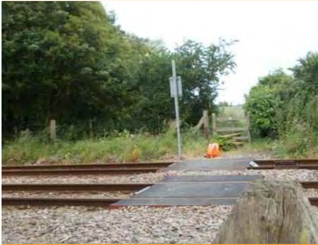
Figure 9.35 Current Saxmundham level crossing (ID SWC47)
