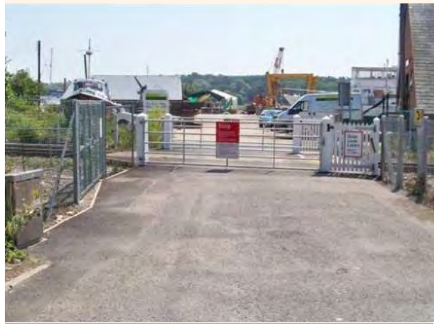
Figure 9.64 Current Dock Lane level crossing (ID SWC21&22)
