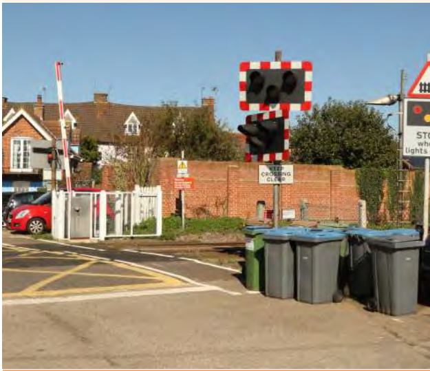
Figure 9.41 Current Ferry Quay level crossing (ID SWC15)
