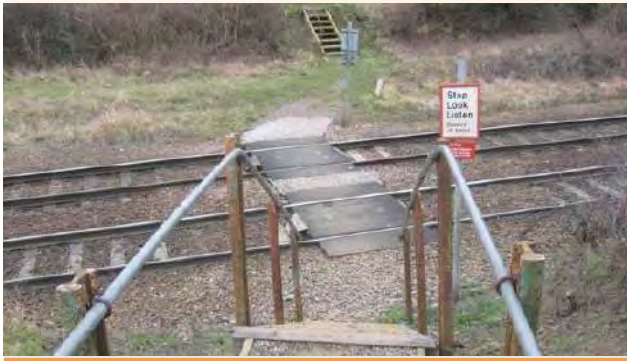
Figure 9.1 Current Westfield footpath level crossing (ID SWC01)
