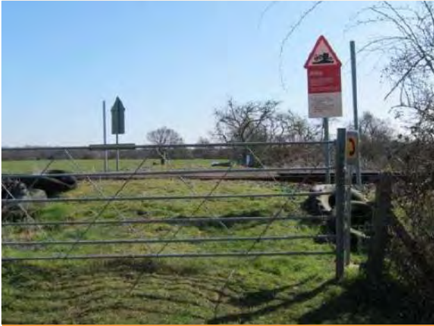
Figure 9.68 Current Uffold level crossing (ID SWC29)
