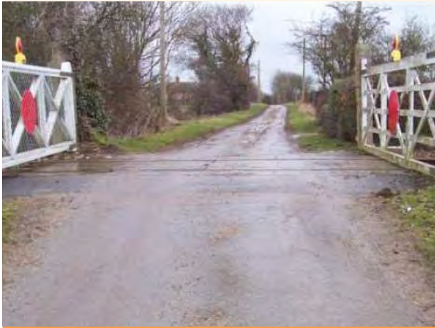
Figure 9.78 Current West House level crossing (ID SWC50)
