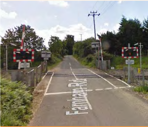
Figure 9.54 Current Beversham level crossing
