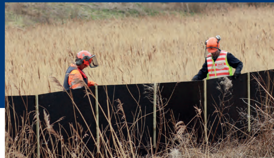
Maintenance being carried out at Aldhurst during March
