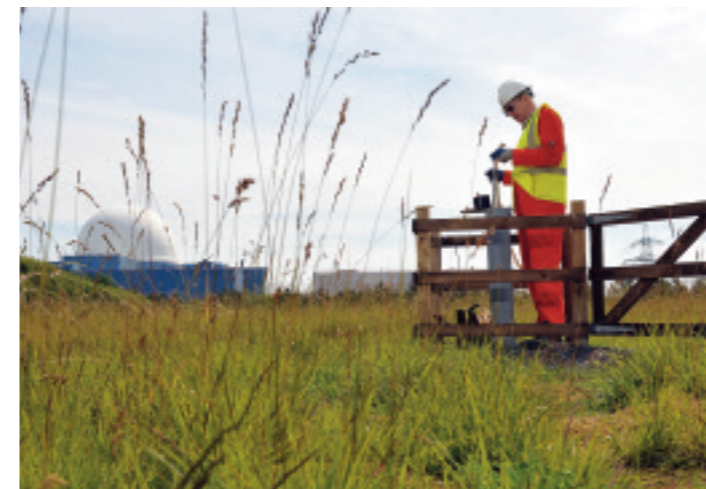
Hydrogeological surveys taking place on the site
