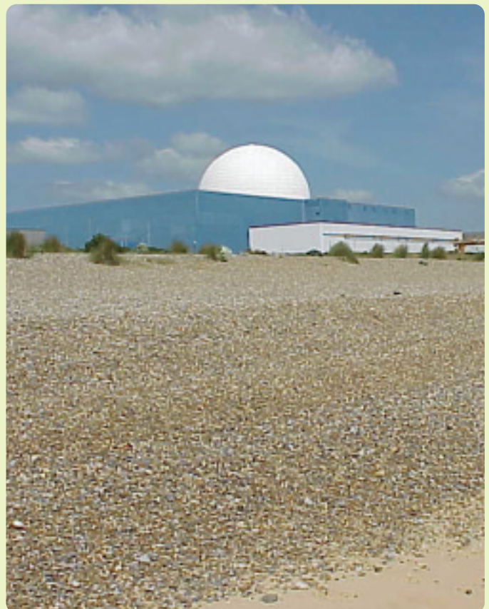
View of Sizewell B power station from the beach
