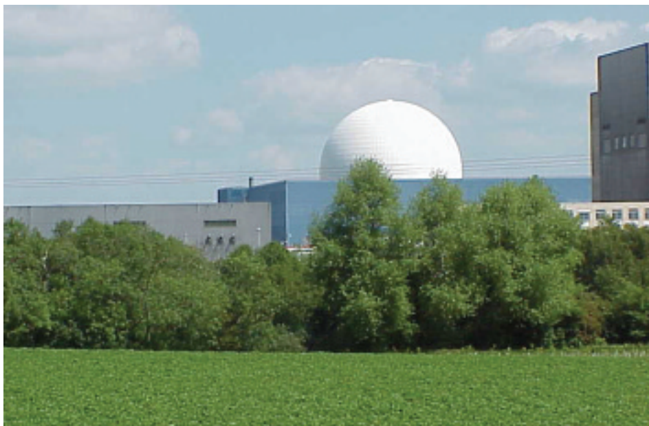
View of Sizewell B. The proposed Sizewell C site is to the north of this station
