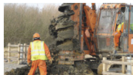
Borehole research work taking place
