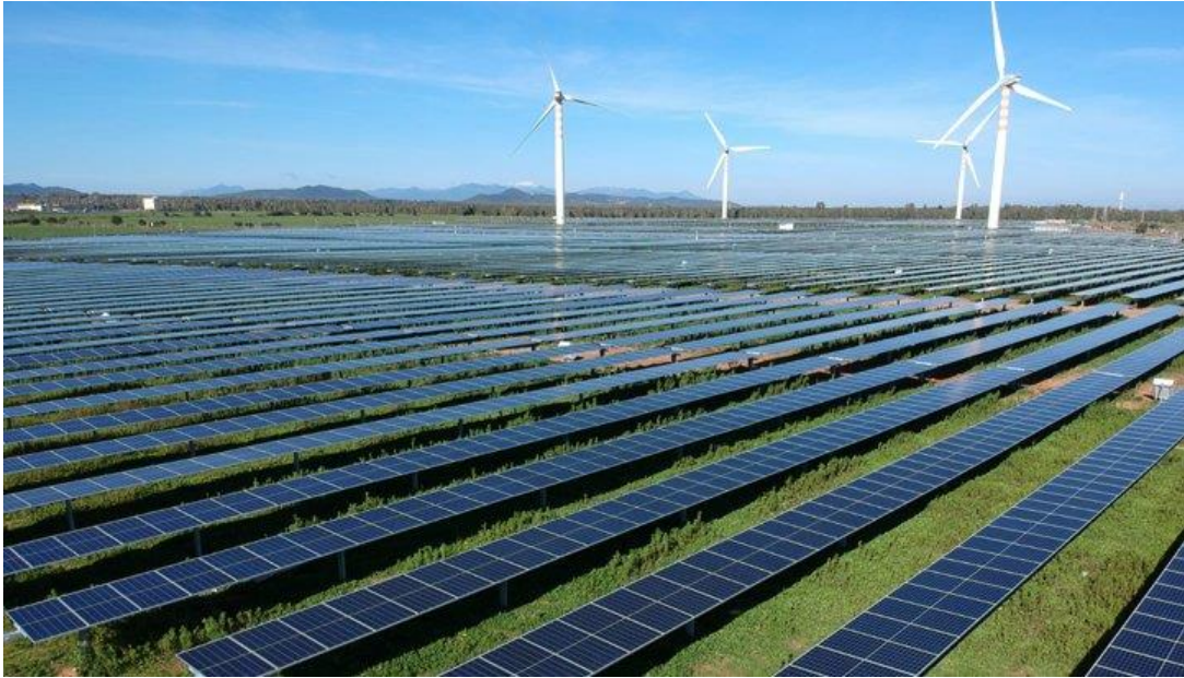
Plate 2: Single Axis Tracker Arrays
