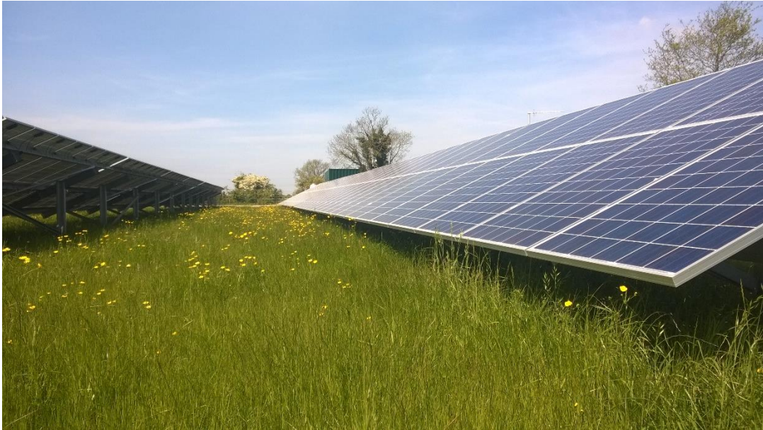
Plate 1: Fixed South Facing Arrays
